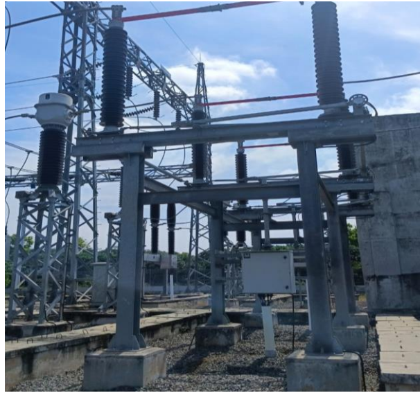
Gambar 3.3 Disconnecting Switch With Earth (Sumber : Dokumentasi, 2024)
