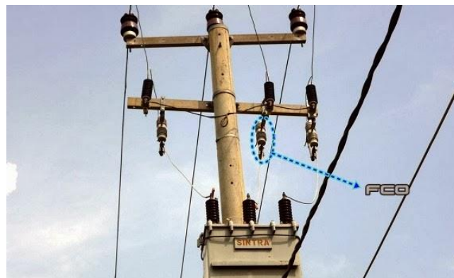
Gambar 3. 7 Fuse Cut Out Sumber: (Google, 2024)
