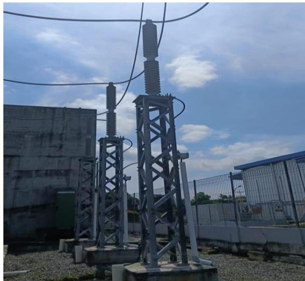
Gambar 3.1 *Lightning Arrester*
