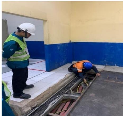
Gambar 2.6 Pemasangan Netral Grounding Trafo
