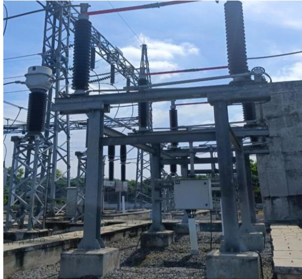
Gambar 3.3 *Disconnecting Switch With Earth (DS/E)*
