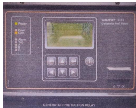
Gambar 3. 9 Modul Relay Proteksi Vamp 210i
