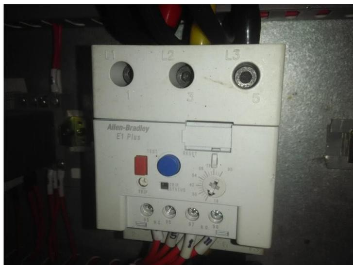
Gambar 3.9 Thermal Over Load Relay (TOLR)
