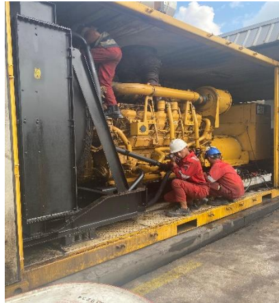
Gambar 4.4 Proses penambahan air radiator
