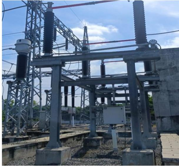
Gambar 3. 3 *Disconnecting Switch With Earth*
