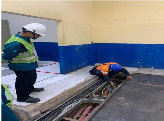
Gambar 2. 6 Pemasangan Netral Grounding Trafo
