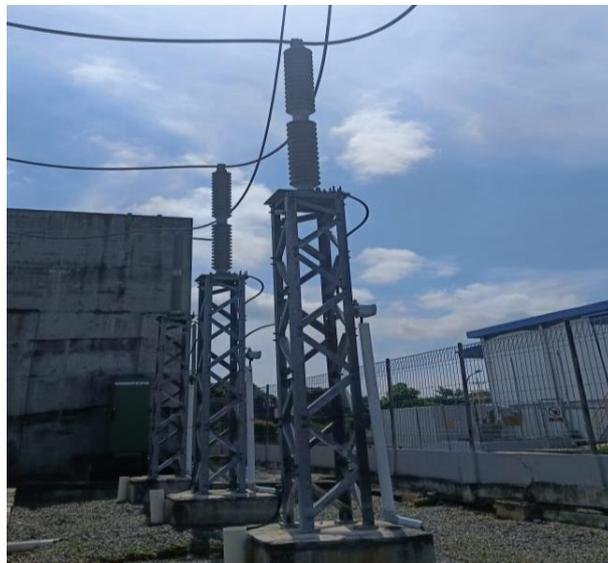
**Gambar 3. 1 Lightning Arrester**
