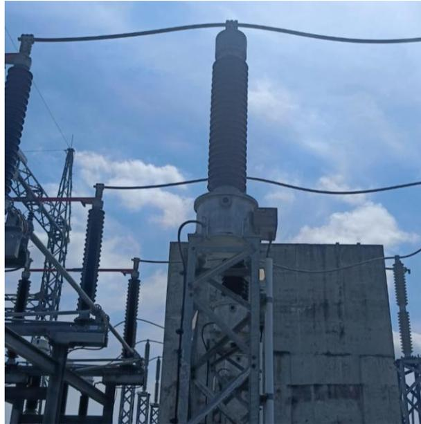
Gambar 3. 2 *Capasitif Voltage Transformer*
