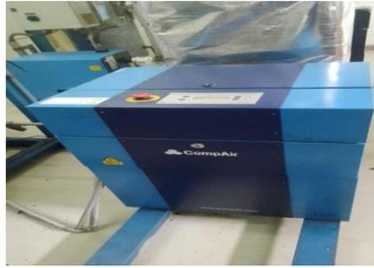
**Gambar 3. 7 Instrumen Air Compressor**
