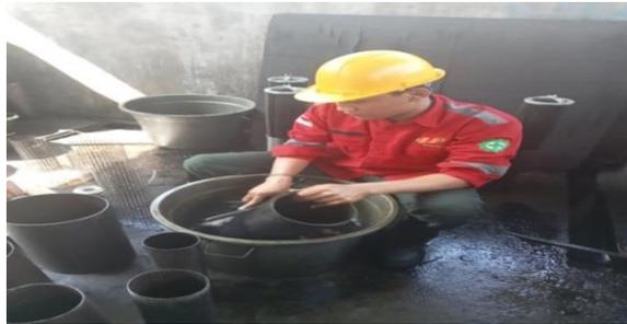
**Gambar 2. 18 Cleaning Filter booster,alo dan insert**
