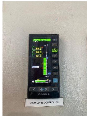
Gambar 3. 5 Drum level controller Sumber : (PT. Kreasijaya Adhikarya)
