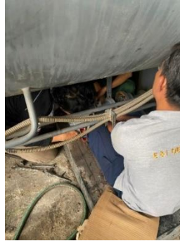
Gambar 2. 27 Melepas refrigerant pump chiller A fractination Sumber : (Dokumentasi, 2024)
