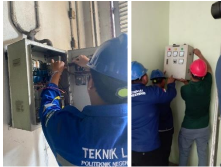
Gambar 2. 45 Move And Replace Lighting Panel Sumber : (Dokumentasi, 2024)
