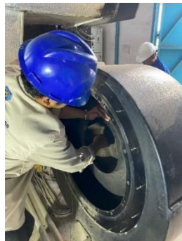
Gambar 2. 21 Proses Cleaning Blower Boiler Sumber : (Dokumentasi, 2024)
