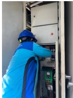
Gambar 2. 18 Cleaning Panel MCC Cooling Tower Sumber : (Dokumentasi, 2024)
