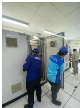
Gambar 2. 19 Cleaning Panel DCS Sumber : (Dokumentasi, 2024)
