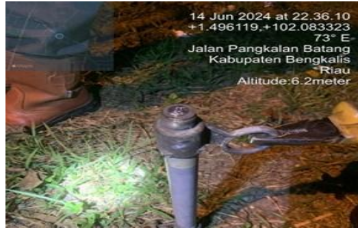
Gambar 2. 9 Penggantian fuse link CO (cut out )
