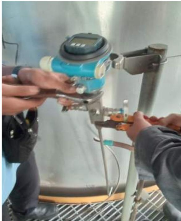
*Gambar 2.5 Mengganti Alat Ukur Pressure*
