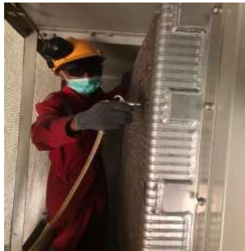
Cleaning Saringan turbin
