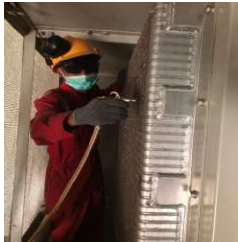
Cleaning Saringan turbin
