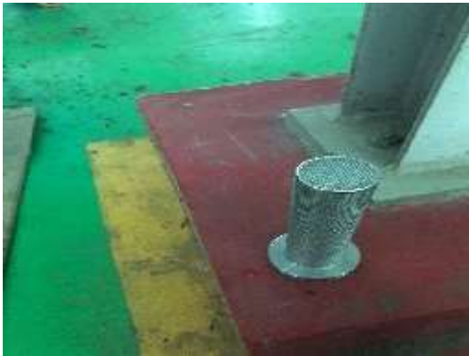
Lanjutan Peggantian Filter Solar
