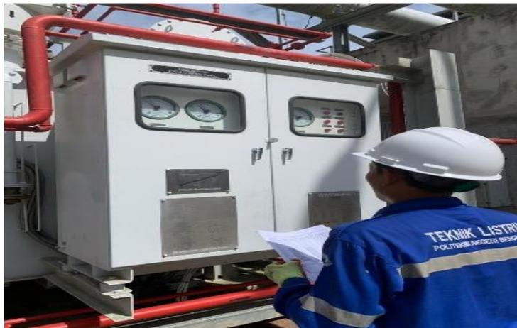
**Gambar 2. 22 Pengecekan Temperature dibagian Transformator**
