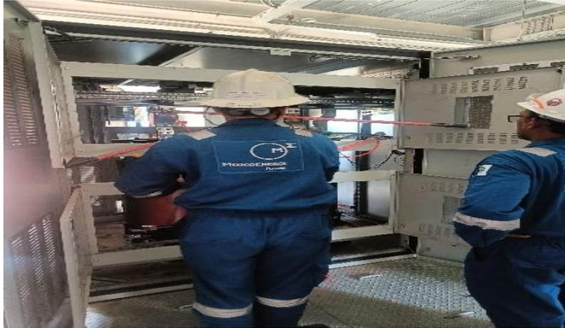
**Gambar 2.23 Pengukuran Insulation Tester di Bagian Trafo Distribusi**
