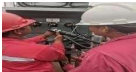
Gambar 2. 14 Termination Kabel
