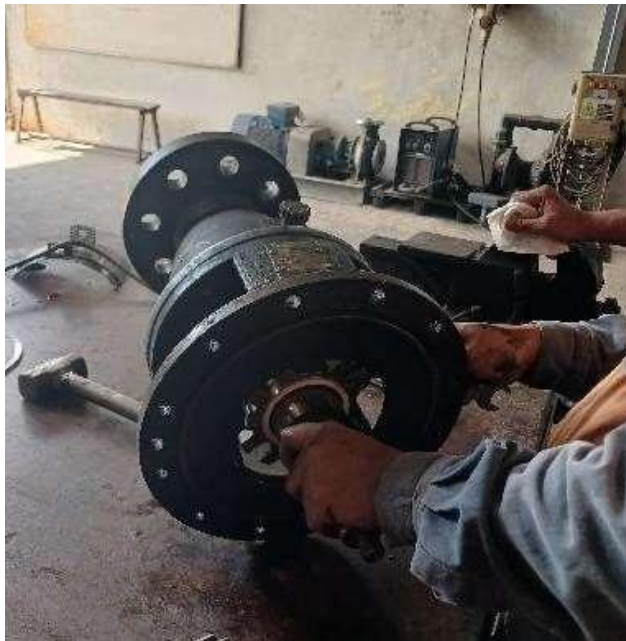
Gambar 4. 11 Pembongkaran mechanical seal cartridge
