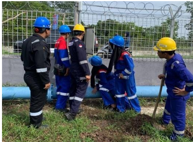
Gambar 3.3 Pemasangan Grounding di Area Marine
