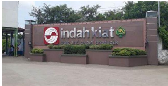
Gambar 2.1 PT. Indah Kiat Pulp & Paper Products Sumber. Data Dokumen PT. Indah Kiat Pulp & Paper Products
