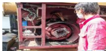
Gambar 2. 58 Servis Genset Sumber: Data Olahan 2024
