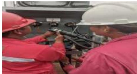
Gambar 2. 14 Termination Kabel Sumber: Data Olahan 2024
