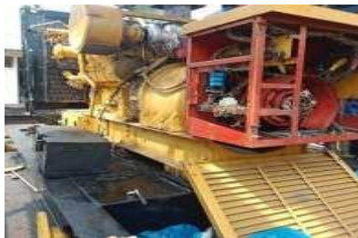
Gambar 2. 29 Servis Genset Sumber: Data Olahan 2024
