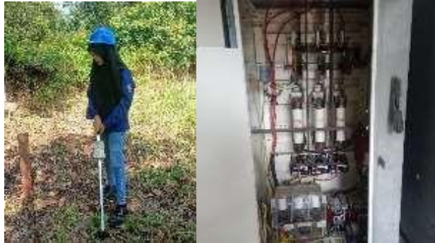
Gambar 2. 3 Check Cable Underground
