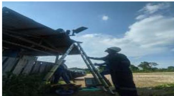
Gambar 2. 16 Install Lighting Sumber: Data Olahan 2024
