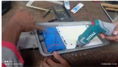
Gambar 2. 53 Install Lampu LED Sumber: Data Olahan 2024
