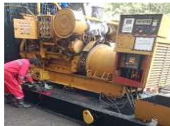
Gambar 2. 22 Setting Speed Control Sumber: Data Olahan 2024
