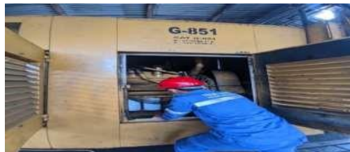
Gambar 2. 6 Prepare Engine Caterpillar
