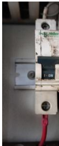
Gambar 3. 6 Miniature Circuit Breaker
