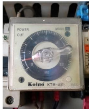
Gambar 3. 13 Time Delay Relay
