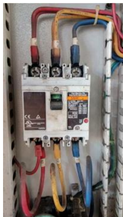
Gambar 3. 5 Case Circuit Breaker
