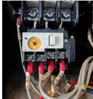
Gambar 3. 12 Thermal Overload Relay
