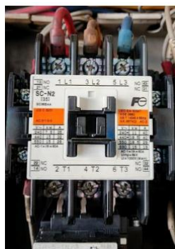
Gambar 3. 7 Magnetic Contactor
