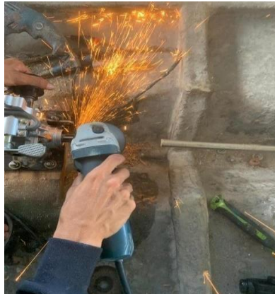
Gambar 4. 17 Pemasangan As Propeller
