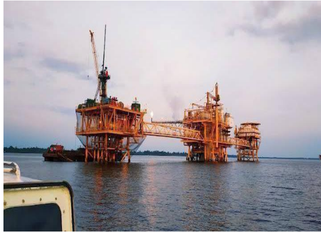
Gambar 2.3 Well Lalang Platform Sumber:PT.Imbang Tata Alam
