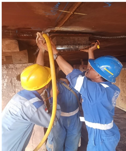
Gambar 2.75 Vacuum Test
