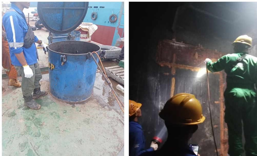
Gambar 2.49 Air Test Wing tank
