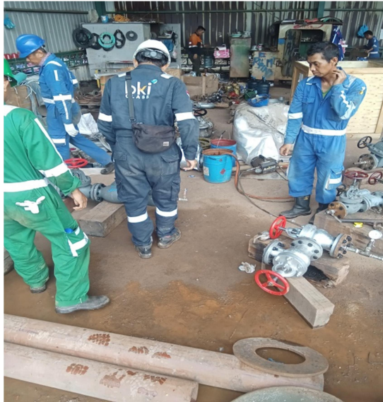
Gambar 2.94 Hydro Test Valve H-075
