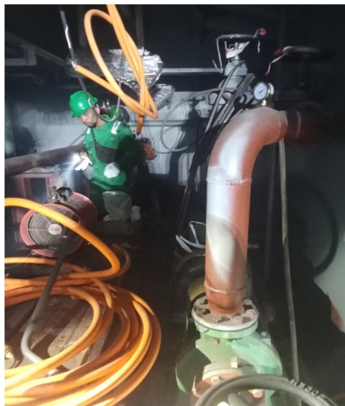
Gambar 2.73 Hydro Test pipa fire
