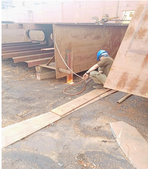
Gambar 2.68 Leveling maindeck wing tank
