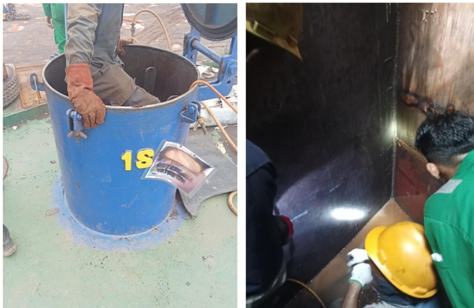
Gambar 2.47 Air Test Wing Tank
