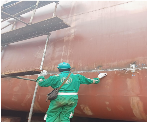
Gambar 2.8 Visual Welding Inspection side shell
