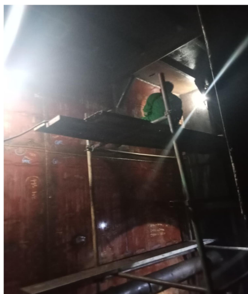
Gambar 2.51 Wing tank 3 port
