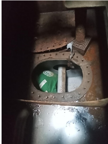
Gambar 2.54 Inspection Double Bottom
