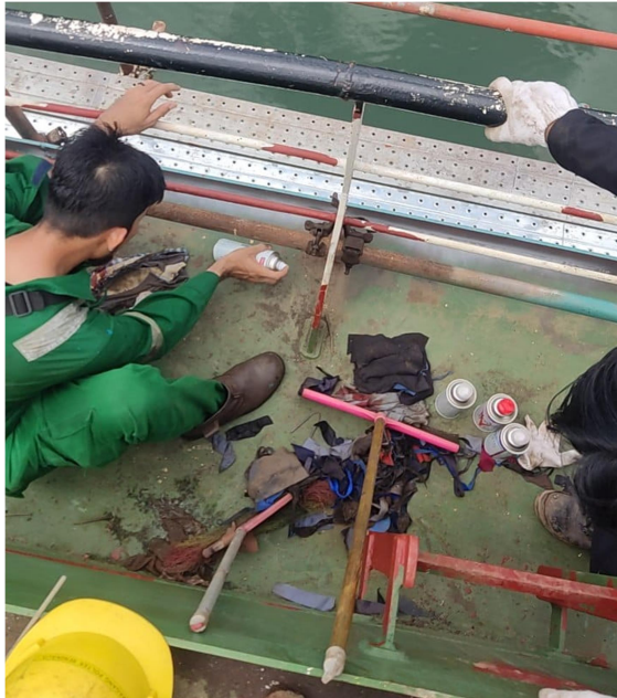
Gambar 2.92 Penetrant Test Insert Plate
