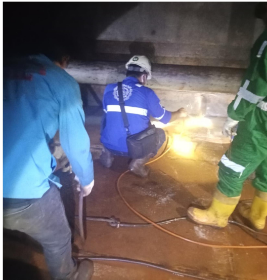
Gambar 2.108 Air Test Tanktop 4 port
