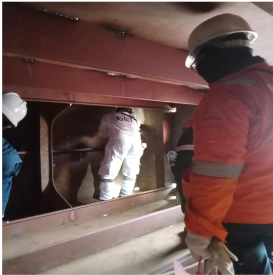
Gambar 2.6 Visual Welding Inspection
