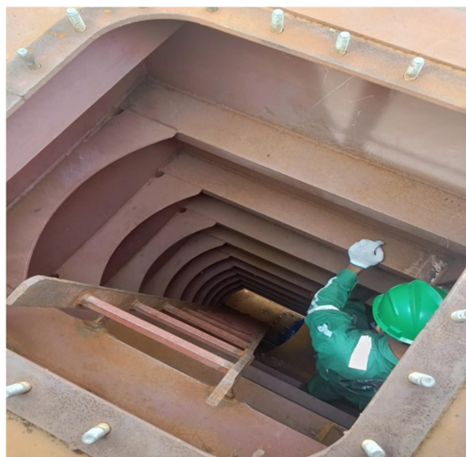
Gambar 2.109 Wing Tank 2 Port
