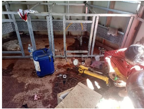
Gambar 2. 37 Hydraulic pressure test di hull 35
