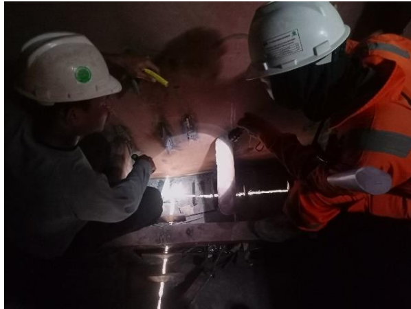
Gambar 2. 9 Inspeksi tangki forepeak hull no 24
