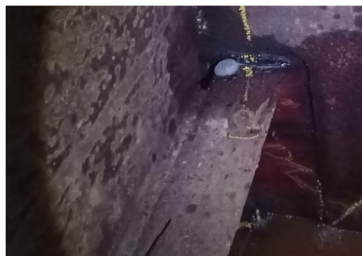
Gambar 3. 22 Area bocor
