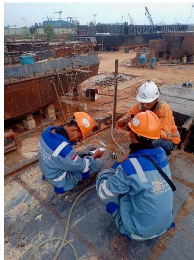
Gambar 2. 5 Leveling raised deck
