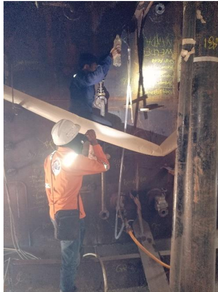
Gambar 2. 36 Air Pressure test tangki Fresh Water hull 38
