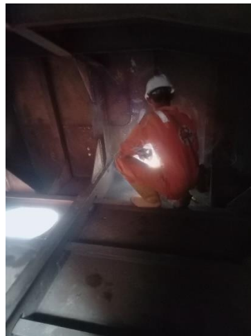
Gambar 2. 18 Visual welding inspection Tank tugboat
