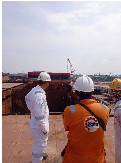
Gambar 2. 26 Pengecekan Progres hull 15
