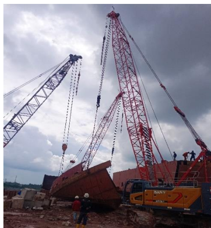
Gambar 2. 8 Erection forepeak barge no 24
