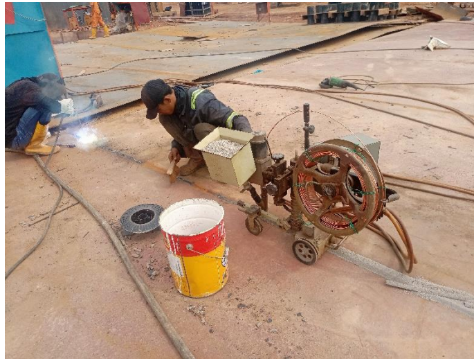
Gambar 2. 7 visual welding inpection (SAW)
