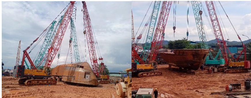
Gambar 2. 49 Lifting turning TB hull 55
