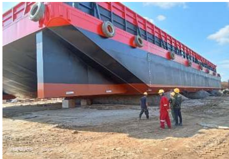
Gambar 2.55 Monitoring Proses Launching Tongkang PSI 2401
