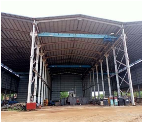
Gambar 1.3 Main Workshop Fabrication
