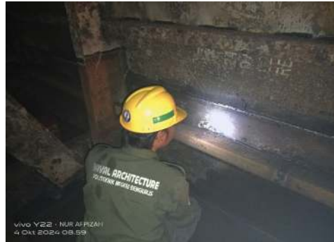
Gambar 2.60 Welding Inspection Tangki 5 Starboard Side Shell
