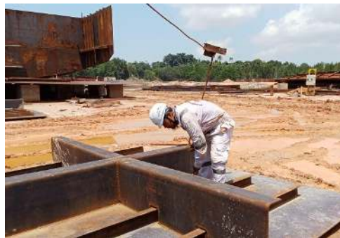
Gambar 2.76 Welding Inspection Tongkang Pelawan Bay 2332
