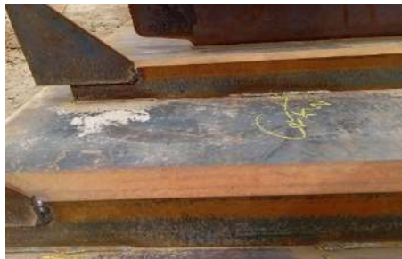
Gambar 2.21 Welding Inspection Skeg,Main Deck dan Bottom Shell Tongkang Makassar Bay
