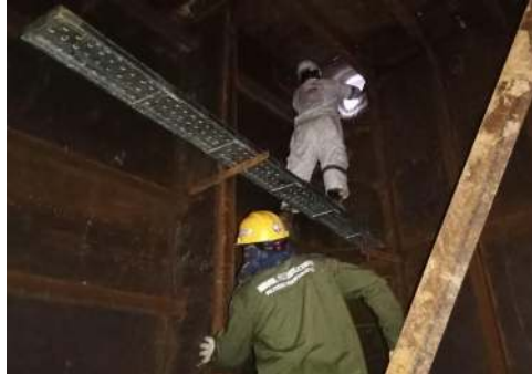
Gambar 2.77 Welding Inspection Tongkang GMS MT 11
