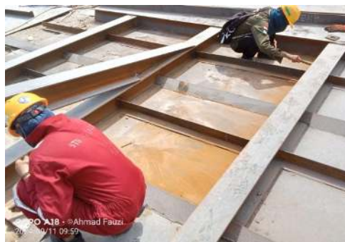
Gambar 2.45 Welding Inspection Side Board Wakatobi Bay 2335
