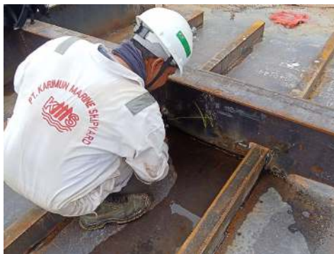
Gambar 2.83 Welding Inspection Tongkang Wakatobi Bay 2336
