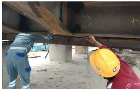
Gambar 2.39 Inpection Welding Rampdoor Tongkang Lantic Bay 1506
