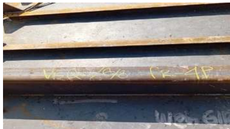
Gambar 2.19 Welding Inspection Transversal Bulkhead Tongkang Manado Bay 2337
