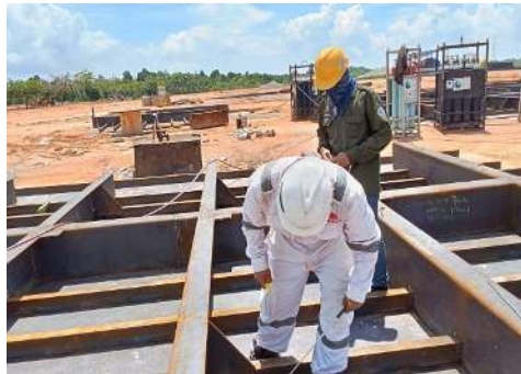
Gambar 2.67 Welding Inspecton Bottom frame 0-6 S Tongkang Tomini Bay 2338
