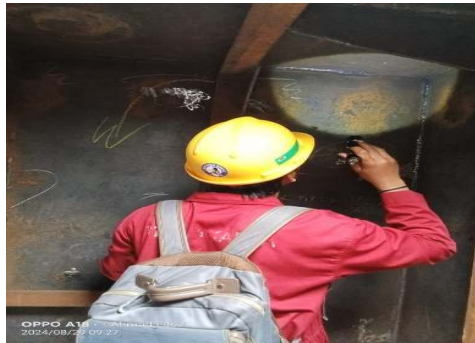
Gambar 2.36 Inspection Welding Winch House Tongkang PSI 2401
