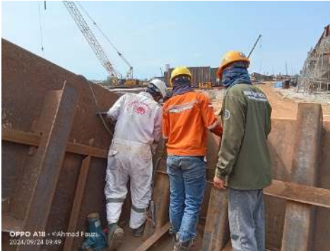
Gambar 2.52 Welding inspection Bottm Stern log Tongkang Wakatobi Bay 2335
