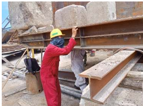
Gambar 2.82 Welding Inspection Rampdoor Nottawasaga Bay 3003
