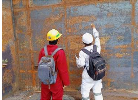
Gambar 2.46 Welding Inspection Seam Joint Long Bhd Wakatobi Bay 2335
