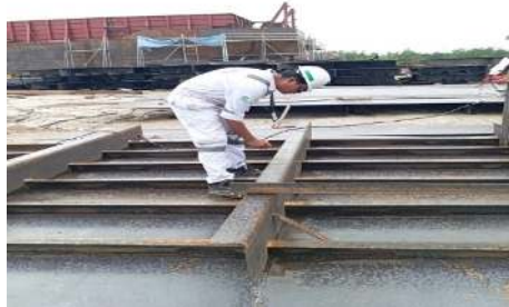
Gambar 2.22 Welding Inspection Transversal Bulkhead Tongkang Manado Bay 2337
