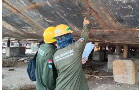
Gambar 2.48 Inspection Welding Seam Joint Bottawasaga Bay 3001
