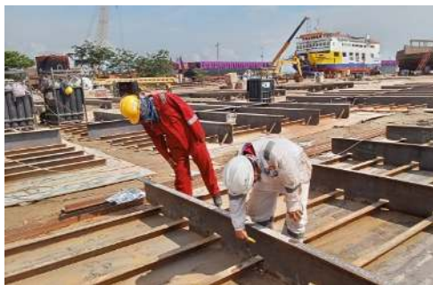
Gambar 2.74 Welding Inspection Tongkang Pelawan Bay 2332
