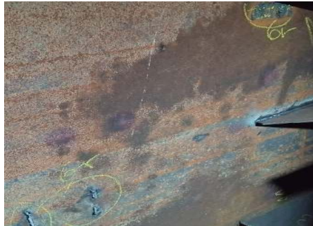
Gambar 2.14 Welding Inspection Tangki Kepala Tongkang Liverpool Bay 2334
