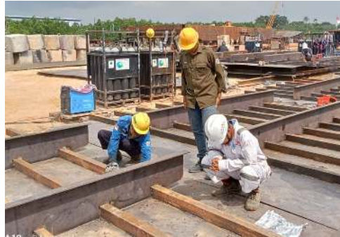
Gambar 2.75 Welding Inspection Main Deck Tongkang 193 GMS MT 11
