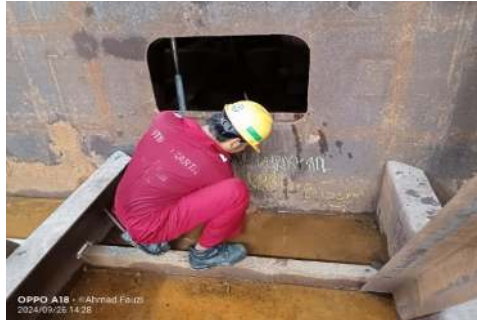
Gambar 2.54 Welding Inspection Tangki 8 bagian Long Bulkhead fr 6-18
