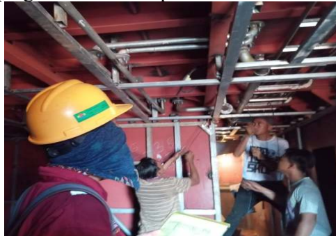
Gambar 2.28 Visual Inspection Piping Gorontalo Dolphin
