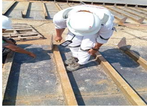
Gambar 2.30 Visual Test Transversal Bulkhead S/CS Manado Bay 2337
