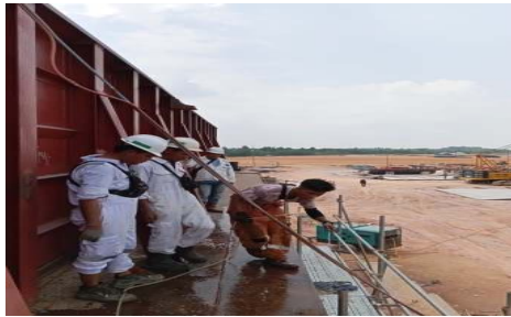
Gambar 2.10 Air Test Tongkang Mamuya Bay 2332
