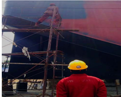
Gambar 2.40 Monitoring Painting Tongkang Halmahera Bay 3004
