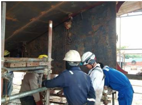
Gambar 2.81 Recheck Bracket,Pipa dan Skeg Tug Boat Chilean Dolphin
