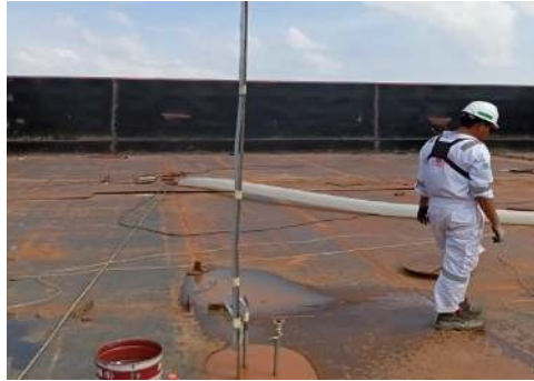
Gambar 2.62 Air Test Tongkang Liverpool Bay 2334
