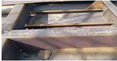
Gambar 2.18 Welding Inspection Longitudinal Bulkhead Tongkang Manado Bay 2335
