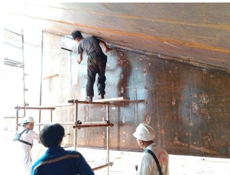
Gambar 2.17 Air Test Skeg Tongkang Mamuya Bay 2332
