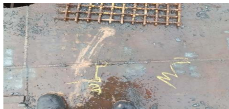
Gambar 2.9 Welding Inspection Tongkang Liverpool Bay 2334
