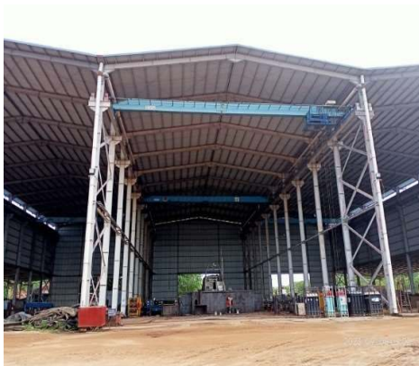
Gambar 1.3 Main Workshop Fabrication
