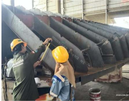
Gambar 2.36 Mengukur bagian double bottom tug boat di Jetty 1
