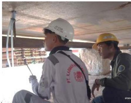
Gambar 2.39 Leveling tongkang H-179
