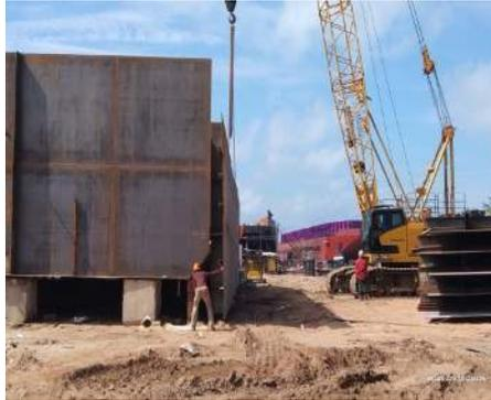
Gambar 2.48 Erection sideshell tongkang
