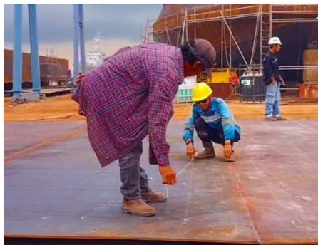
Gambar 2.41 Marking tongkang bottom
