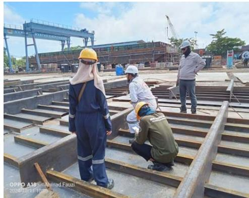
Gambar 3.5.7. Inspection Fit up panel bottom tongkang
