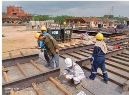
Gambar 2.76 welding inspection
