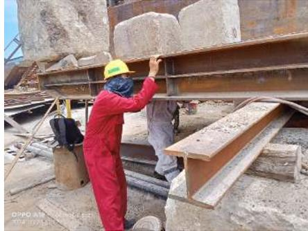
Gambar 2.84 Welding inspection
