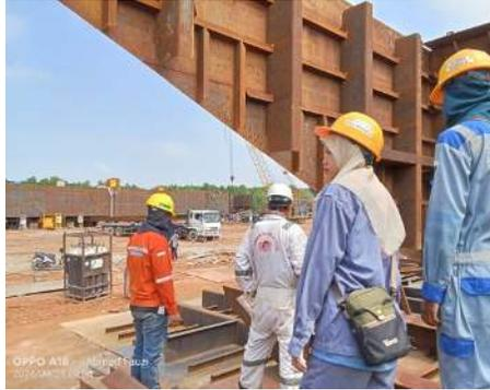
Gambar 2.54 Visual inspection headlog tongkang H-180
