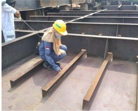
Gambar 2.40 Visual test H-181 main deck
