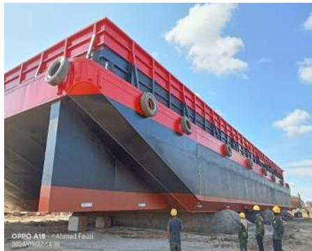
Gambar 2.57 Melihat proses launching tongkang
