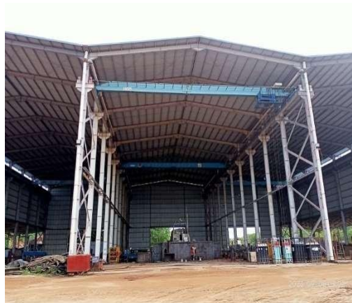
Gambar 1.3 Main Workshop Fabrication
