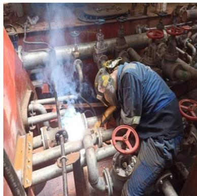
Gambar 2.66 Pengecekan Pemasangan Piping Tugboat
