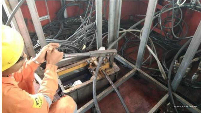
Gambar 3.12. Hand Pump/Hydrolic Pump
