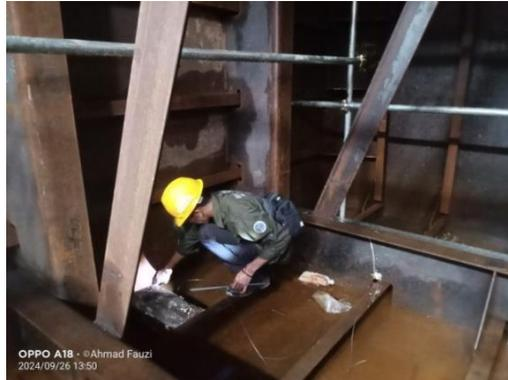
Gambar 2.10 Inspection Welding Long Bulkhead dan Trans Bulkhead
