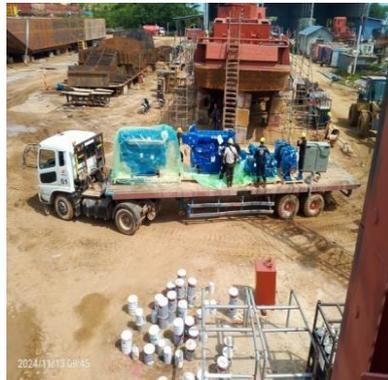
Gambar 2.43 Pengecekan Pemasangan ME, Tugboat Chilean Dolpin
