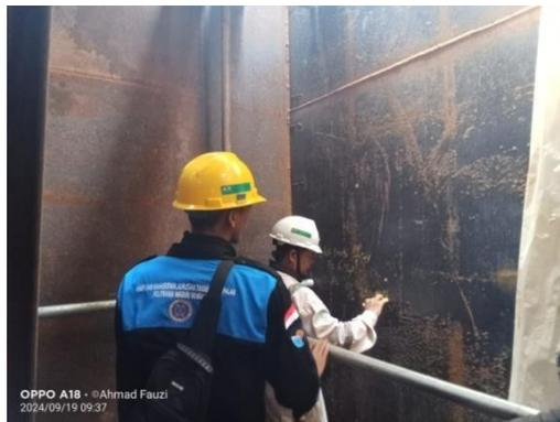
Gambar 2.5 Inspection Welding Long Bulkhead Dan Trans Bulkhead
