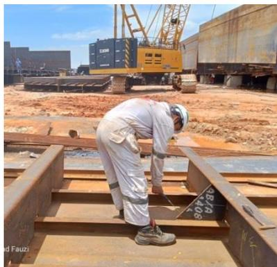
Gambar 2.7 Inspection Welding
