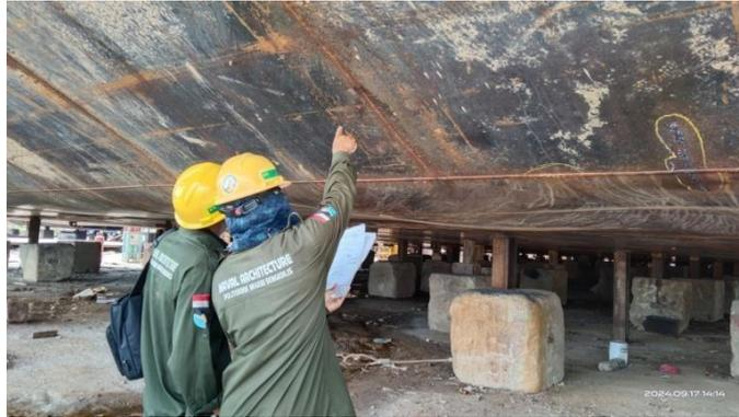
Gambar 2.3 Inspection Welding Seam Joint
