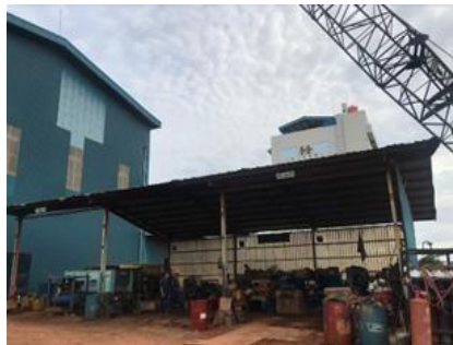
Gambar 1. 9. Workshop Mechanical & Electrical
