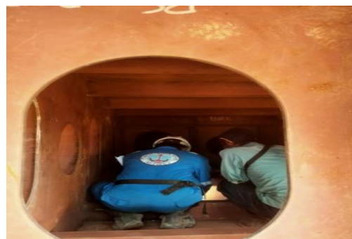
Gambar 2. 7. Visual Weld Inspection Joinant plat Bottom
