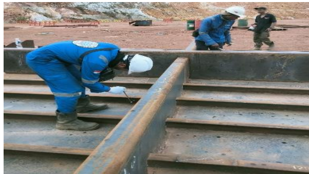
Gambar 2. 128. Visual Weld Inspection
