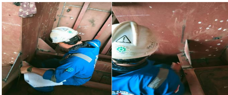
Gambar 2. 221. Fit Up Blok Raised Deck
