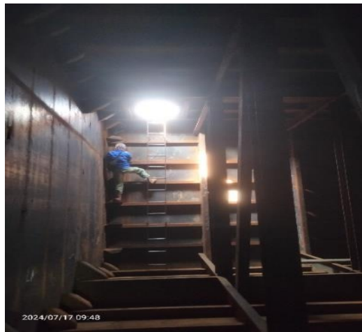
Gambar 2. 20. Visual Weld Inspection Tank
