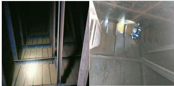
Gambar 2. 130. Final Inspect Tank
