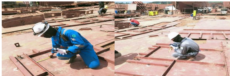
Gambar 2. 174. Fit Up Blok Wheel House
