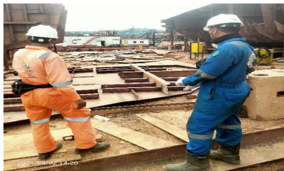
Gambar 2. 57. Visual Weld Inspection T.Bulkhead
