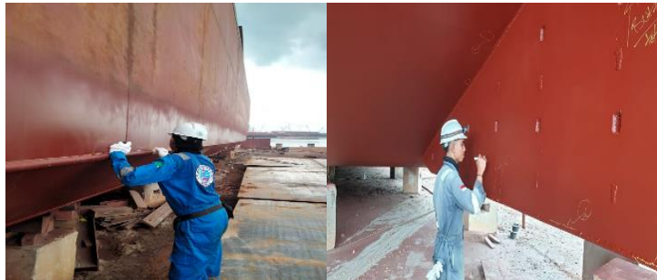
Gambar 2. 241. Visual Weld After Primer Coating
