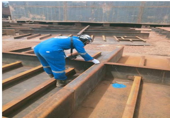
Gambar 2. 190. Visual Weld Inspection Tank
