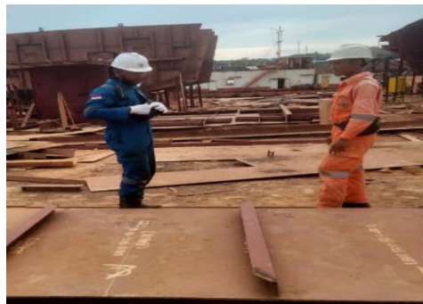
Gambar 2. 60. Fit Up L.Bulkhead
