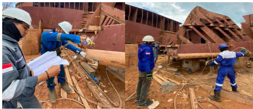
Gambar 2. 153. Levelling Raised Deck
