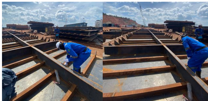
Gambar 2. 151. Visual Weld Inspection T.Bulkhead
