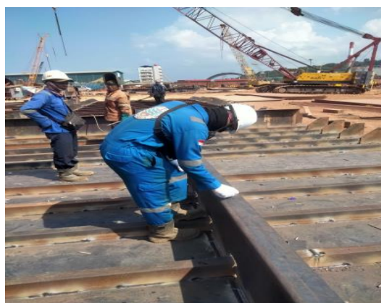
Gambar 2. 46. Visual Weld Inspection T.Bulkhead
