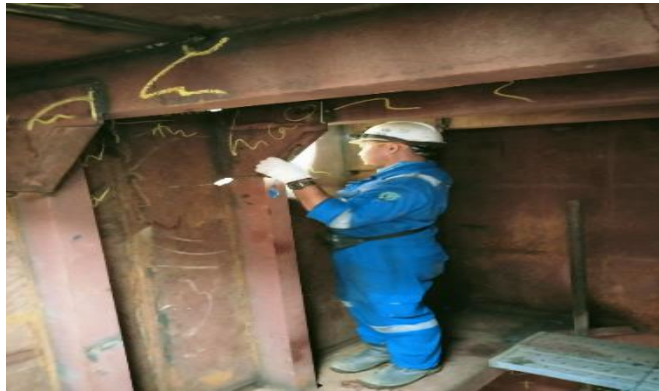
Gambar 2. 160. Visual Weld Inspection Tank
