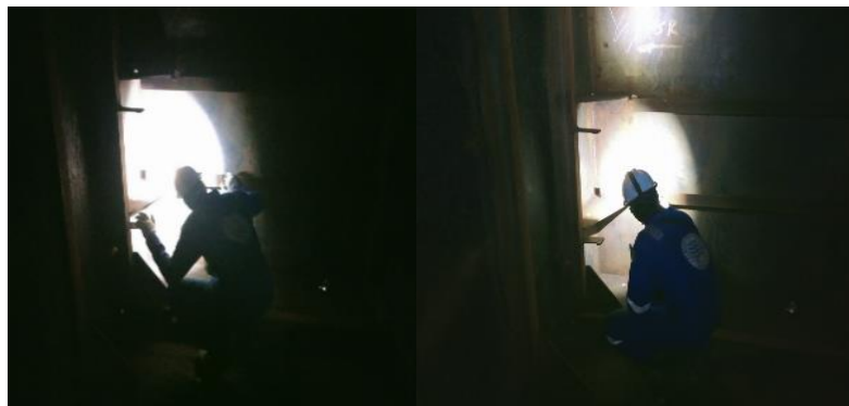
Gambar 2. 201. Visual Welding Inspection Tank
