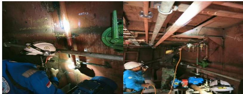
Gambar 2. 218. Air Test and Hydro Test
