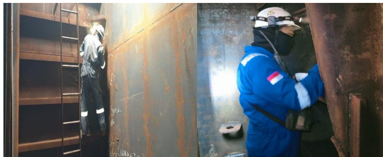
Gambar 2. 213. Visual Welding Inspection
