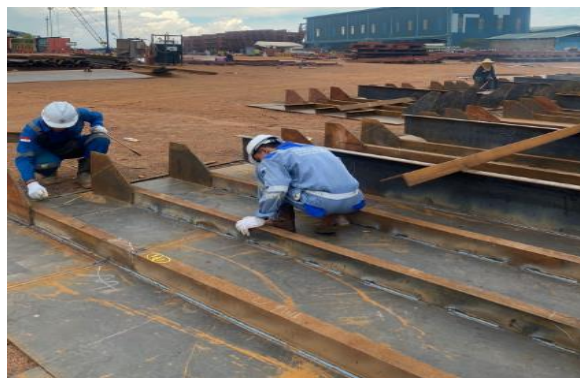
Gambar 2. 100. Visual Weld Inspection T.Bulkhead
