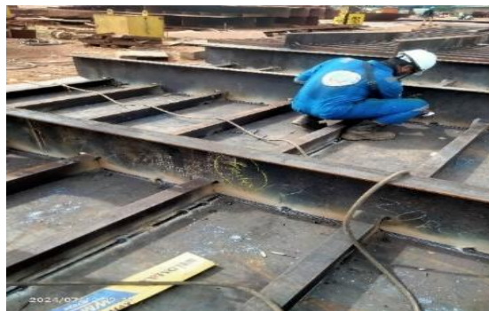
Gambar 2. 11. Fit Up Long Bulkhead
