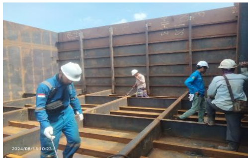
Gambar 2. 85. Visual Weld Inspection With OS LDU
