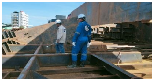
Gambar 2. 129. Visual Weld Inspection
