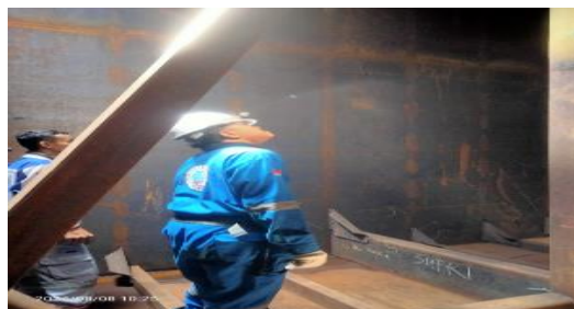
Gambar 2. 71. Visual Weld Inspection Tank
