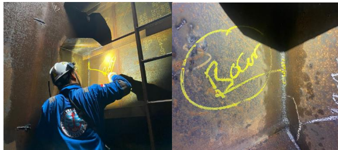
Gambar 2. 136. Air Test Tank
