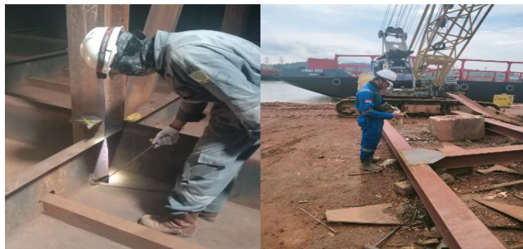
Gambar 2. 220. Visual Welding Inspection
