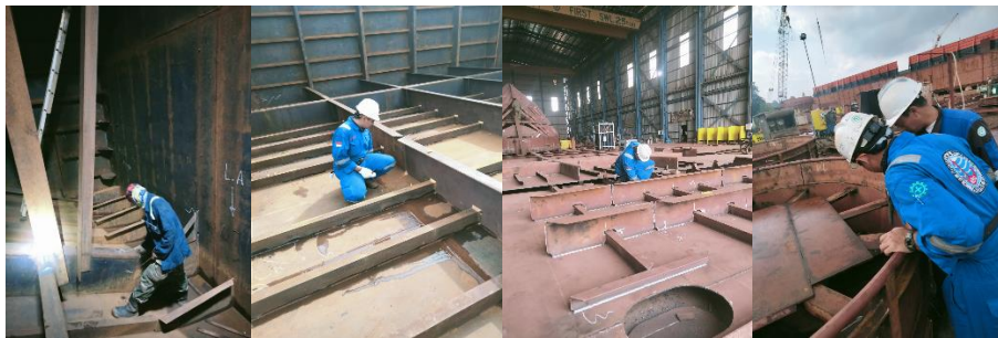
Gambar 2. 227. Visual Welding Inspection
