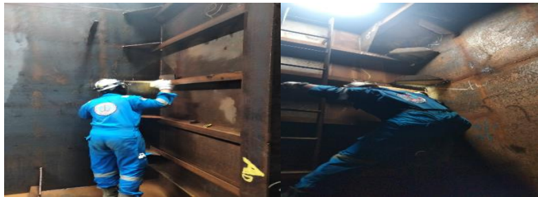
Gambar 2. 236. Visual Welding Inspection Tank
