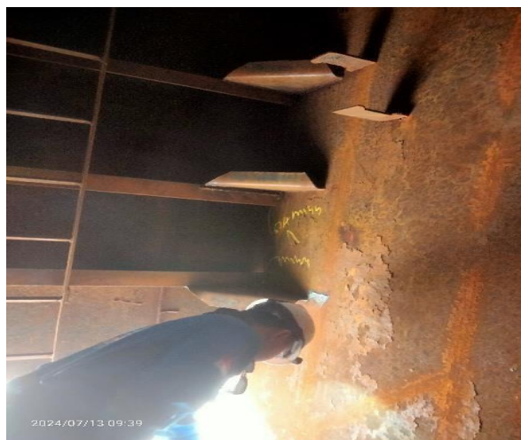
Gambar 2. 13. Visual Welding Inspection
