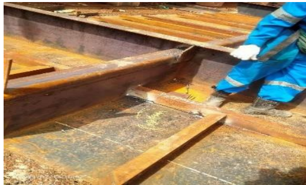
Gambar 2. 14. Visual Welding Inspection
