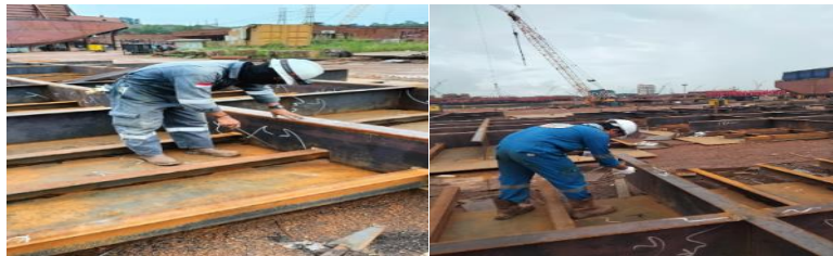
Gambar 2. 234. Visual Welding Inspection
