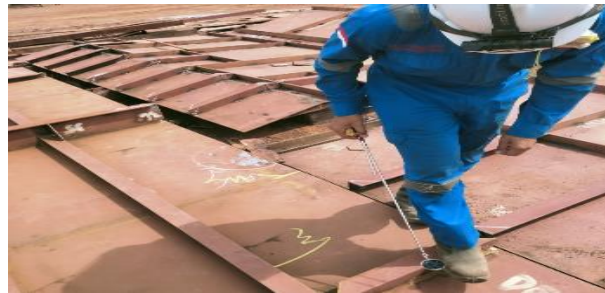
Gambar 2. 176. Visual Weld Inspection
