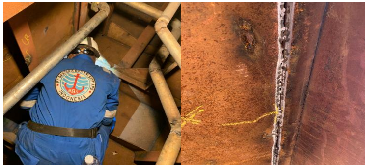
Gambar 2. 134. Visual Weld Inspection Tank Cofferdam
