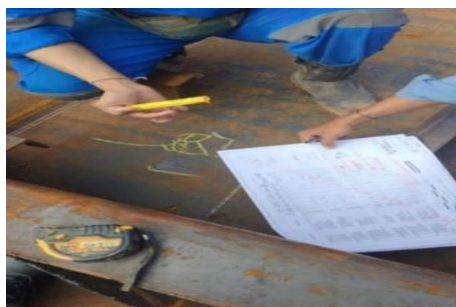
Gambar 2. 5. Visual Weld Inspection Side Shell
