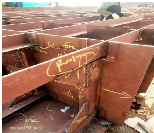
Gambar 2. 34. Visual Weld Inspection Wing Tank
