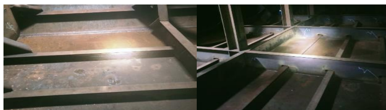
Gambar 2. 219. Final Inspection Tank
