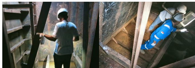
Gambar 2. 162. Final Inspection Tank
