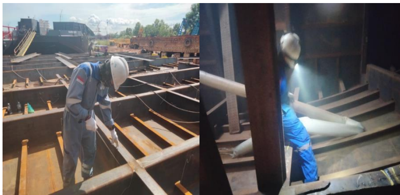
Gambar 2. 252. Visual Welding Inspection
