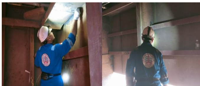
Gambar 2. 161. Visual Weld Inspection Tank
