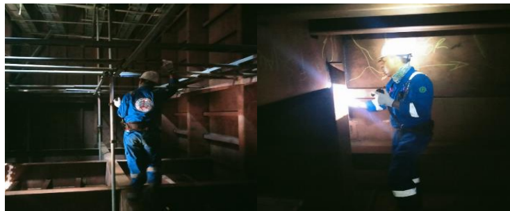
Gambar 2. 188. Visual Weld Inspection Tank
