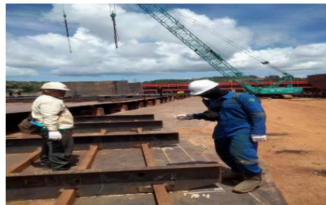
Gambar 2. 61. Visual Weld Inspection L.Bulkhead
