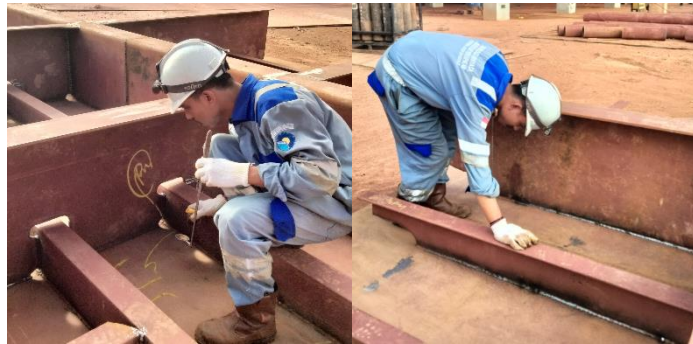
Gambar 2. 146. Visual Weld Inspection Main Deck
