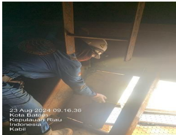
Gambar 2. 102. Fit Up Bracket Chine
