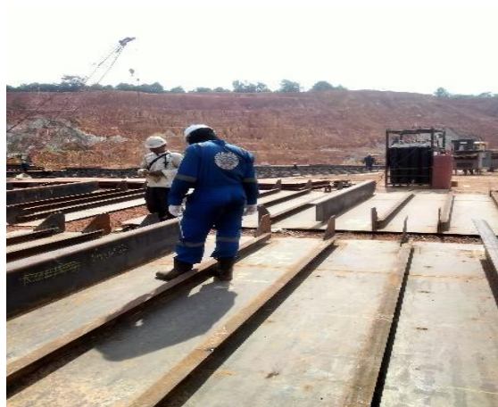
Gambar 2. 38. Visual Weld Inspection T.Bulkhead
