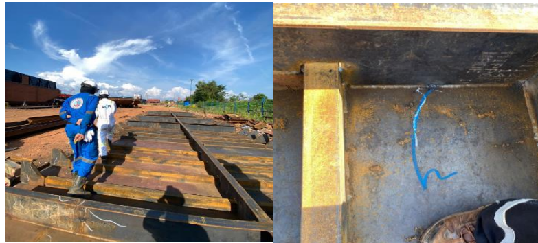
Gambar 2. 170. Visual Weld Inspection with RINA Surveyor
