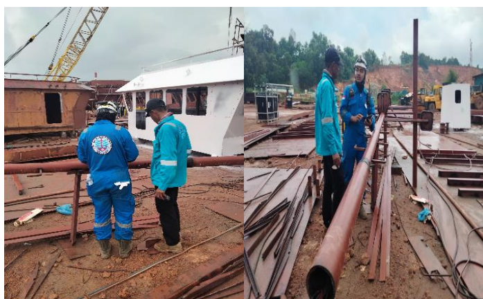
Gambar 2. 244. Scantling Fit Up Tiang Mast
