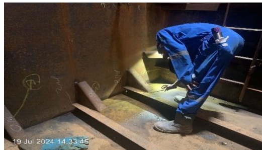
Gambar 2. 26. Visual Welding Inspection Tank
