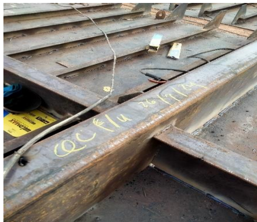
Gambar 2. 41. Fit Up T.Bulkhead
