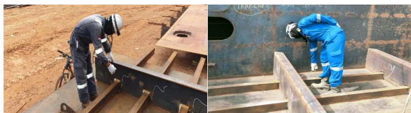
Gambar 2. 209. Visual Welding Inpection
