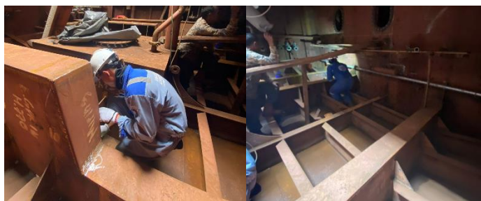
Gambar 2. 131. Visual Weld Inspection Engine Girder
