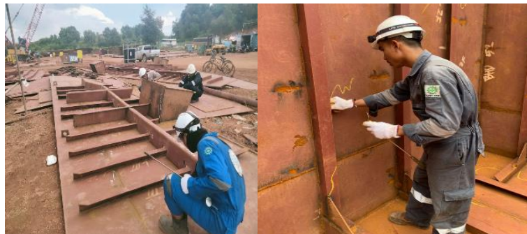
Gambar 2. 187. Visual Weld Inspection
