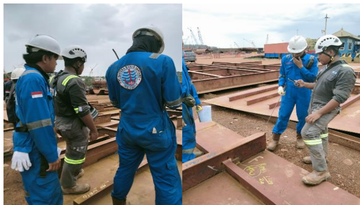
Gambar 2. 175. Visual Weld Inspection With Class
