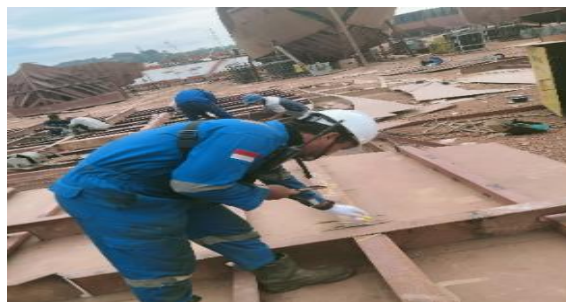
Gambar 2. 148. Fit Up Panel Main Deck
