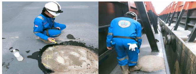
Gambar 2. 172. Cek Kebocoran Manhole
