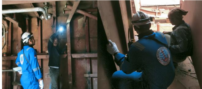
Gambar 2. 154. Fit Up Markingan Sanitary Pipe
