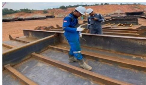
Gambar 2. 110. Visual Weld Inspection
