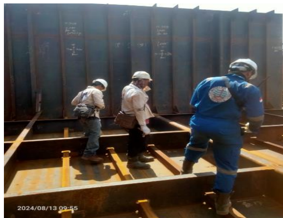
Gambar 2. 80. Visual Weld Inspection With OS LDU
