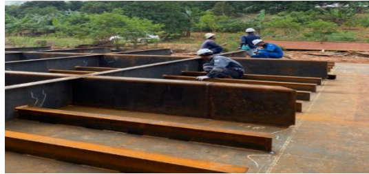
Gambar 2. 109. Visual Weld Inspection
