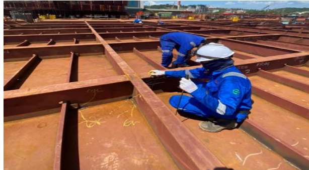
Gambar 2. 99. Visual Weld Inspection
