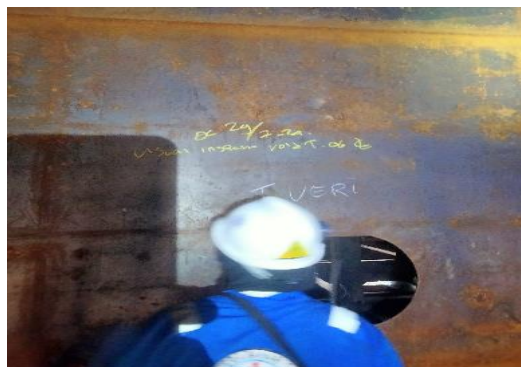
Gambar 2. 53. Visual Weld Inspectio Tank
