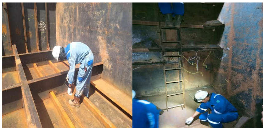
Gambar 2. 256. Visual Welding Inspection Tank and Panel
