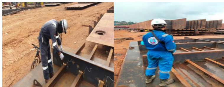
Gambar 2. 233. Visual Welding Inspection
