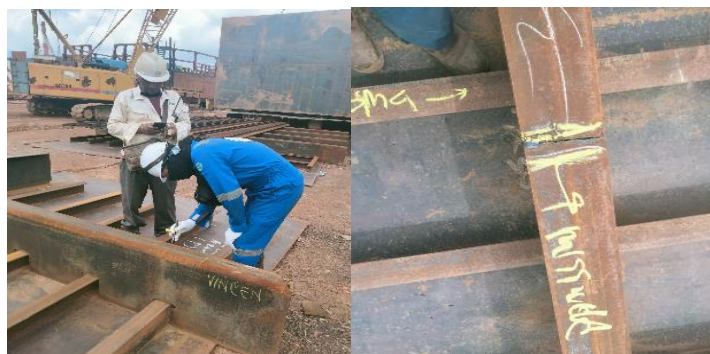
Gambar 2. 185. Visual Weld Inspection
