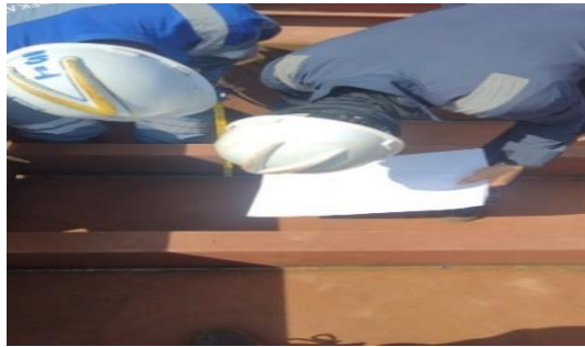
Gambar 2. 10. Visual Weld Inspection Main Deck and Side Shell
