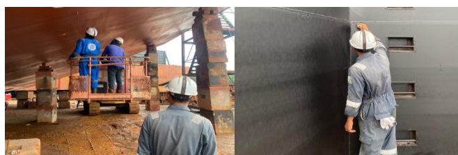
Gambar 2. 149. Final Inspection Eksternal
