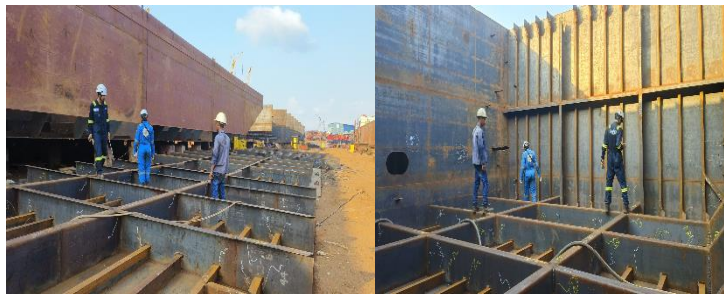
Gambar 2. 113. Visual Weld Inspection with RINA Surveyor
