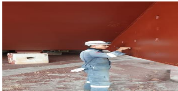
Gambar 2. 240. Visual Weld After Primer Coating
