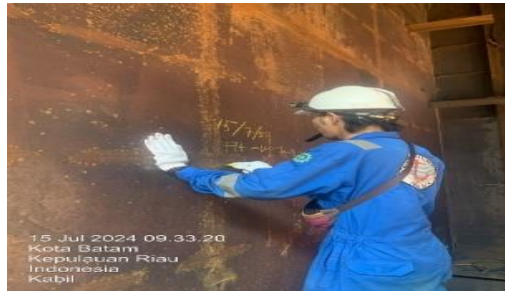
Gambar 2. 16. Fit Up Tank
