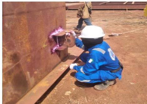
Gambar 2. 96. Penetrant Test kupingan Blok Wing Tank
