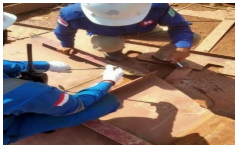
Gambar 2. 6. Visual Weld Inspection Long & Trans Bulkhead Tugboat
