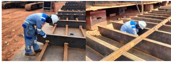
Gambar 2. 147. Visual Weld Inspection
