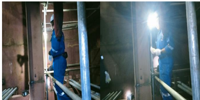
Gambar 2. 165. Visual Weld Inspection Tank
