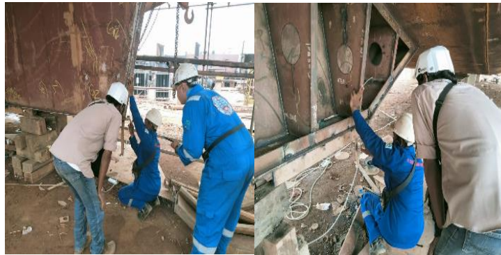
Gambar 2. 204. Levelling Cek Skeg
