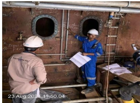
Gambar 2. 104. Fit Up Line Pipe with OS
