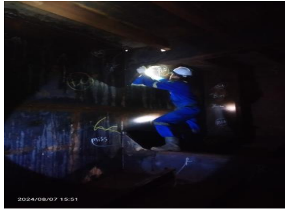
Gambar 2. 70. Air Test Internal Tank
