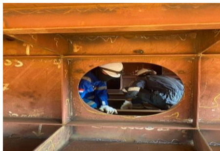
Gambar 2. 93. Visual Weld Inspection Block Wing Tank
