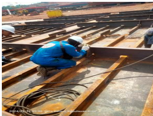
Gambar 2. 27. Visual Weld Inspection L.Bulkhead
