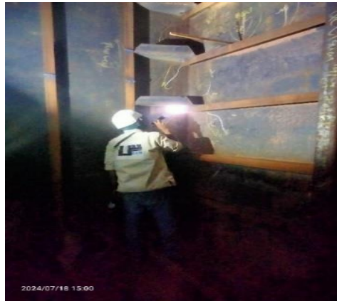
Gambar 2. 24. Visual Welding Inspection Tank
