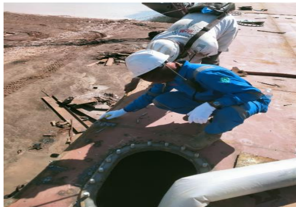
Gambar 2. 179. Visual Weld Inspection
