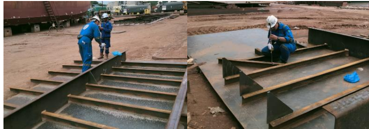
Gambar 2. 166. Visual Weld Inspection
