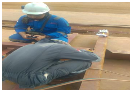
Gambar 2. 77. Visual Weld Inspection
