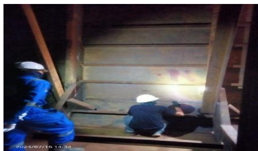
Gambar 2. 17. Visual Welding Inspection Tank
