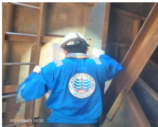
Gambar 2. 59. Visual Weld Inspection Tank
