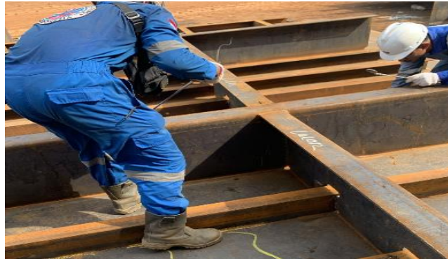
Gambar 2. 116. Visual Weld Inspection
