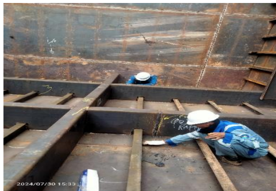
Gambar 2. 50. Visual Weld Inspection Bottom
