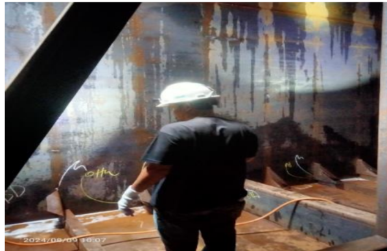
Gambar 2. 73. Air Test Internal Tank
