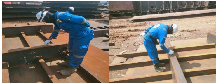
Gambar 2. 197. Visual Welding Inspection
