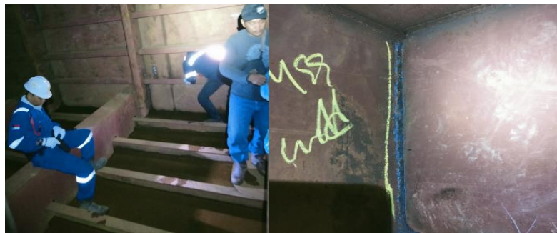
Gambar 2. 158. Visual Weld Inspection Tank
