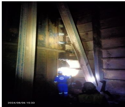
Gambar 2. 67. Air Test Internal Tank
