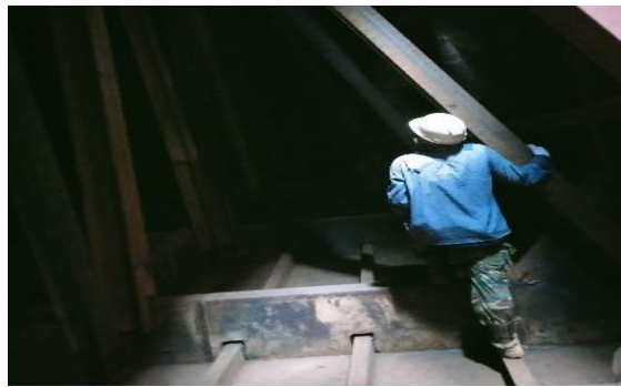
Gambar 2.124. Final Inspect Tank
