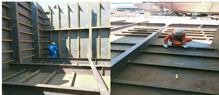
Gambar 2. 225. Visual Welding Inspection
