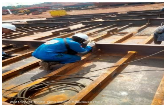
Gambar 2. 9. Visual Weld Inspection Long Bulkhead
