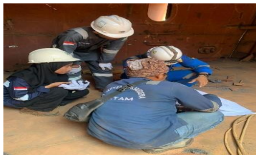
Gambar 2.125. Fit Up Markingan Over Board
