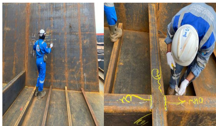
Gambar 2. 157. Visual Weld Inspection Bottom
