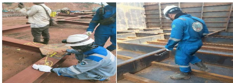
Gambar 2. 224. Visual Welding Inspection
