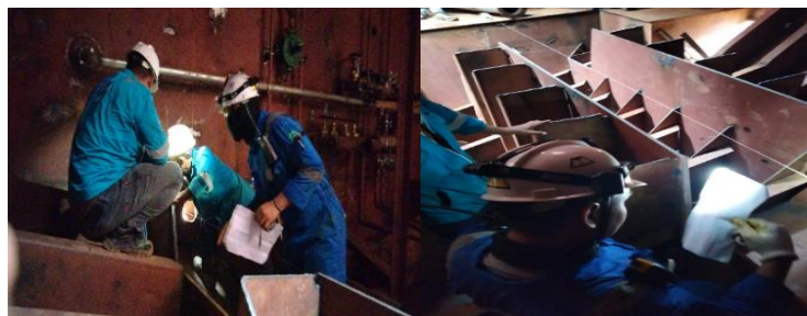
Gambar 2. 239. Fit Up Engine Girder
