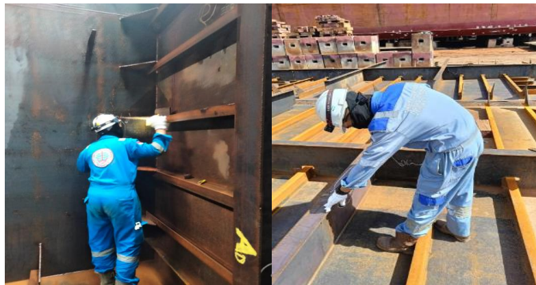
Gambar 2. 257. Visual Welding Inspection
