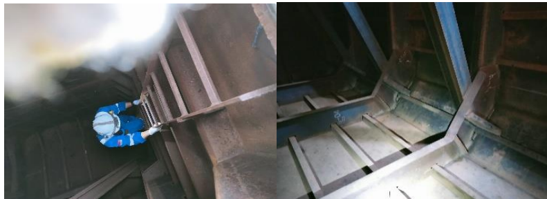
Gambar 2. 132. Final Inspection Tank
