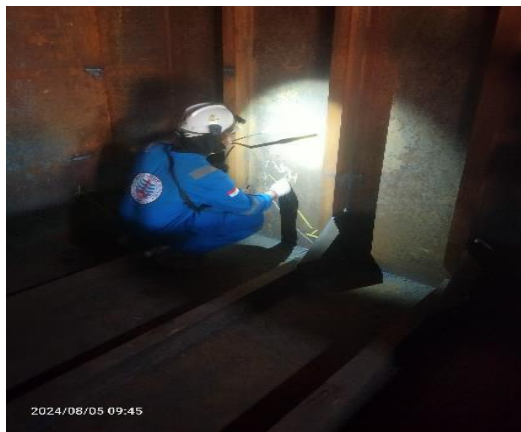
Gambar 2. 62. Visual Weld Inspection Tank
