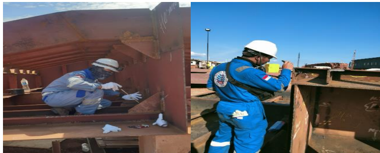
Gambar 2. 223. Visual Welding Inspection
