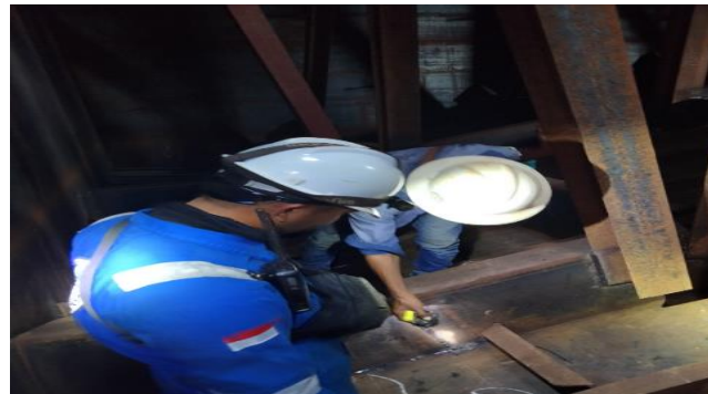
Gambar 2. 247. Visual Welding Inspection Tank
