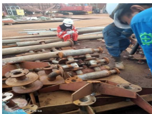
Gambar 2. 69. Visual Weld fabricaton Pipe
