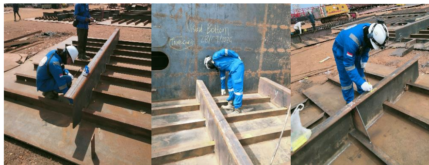
Gambar 2. 203. Visual Welding Inspection
