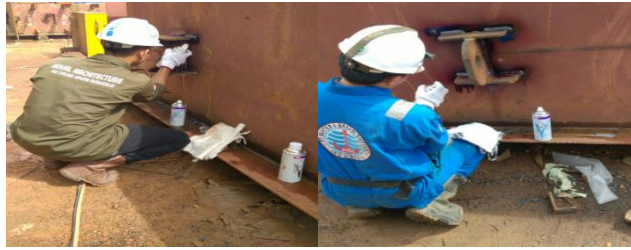
Gambar 2. 75. Penetrant Test kupingan Blok Wing Tank
