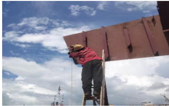
Gambar 2. 94. Levelling T.Bulkhead
