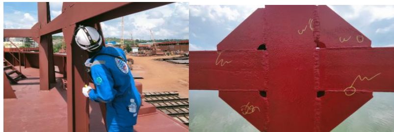
Gambar 2. 178. Final Visual Weld Inspection
