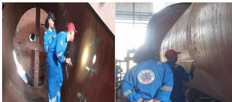
Gambar 2. 137. Survey dan Visual Weld Inspection PEDESTAL
