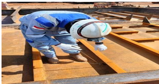
Gambar 2. 243. Visual Welding Inspection
