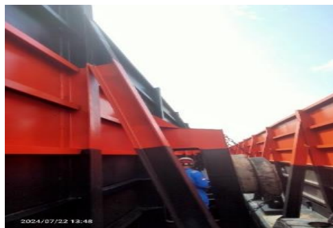
Gambar 2. 29. Final Inspect Painting
