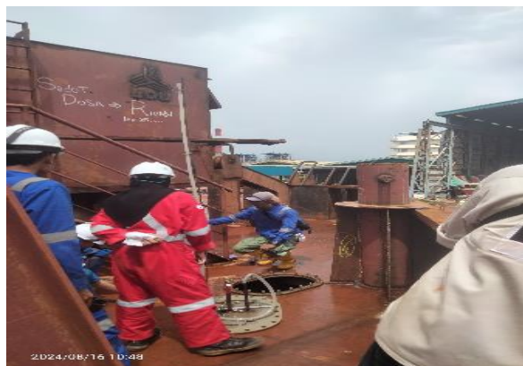
Gambar 2. 89. Visual Weld Inspection Tank With OS LDU
