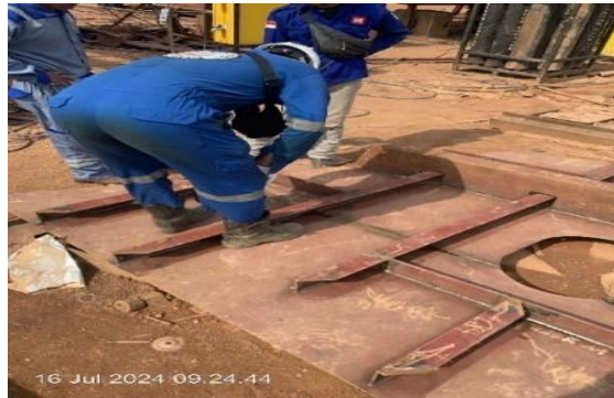
Gambar 2. 18. Visual Weld Inspection T.Bulkhead
