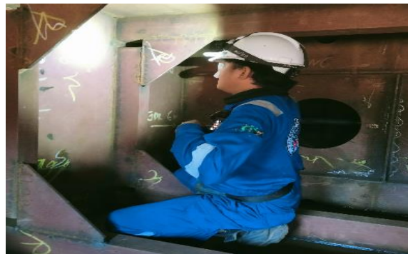
Gambar 2. 144. Visual Weld Inspection Double Bottom Tank
