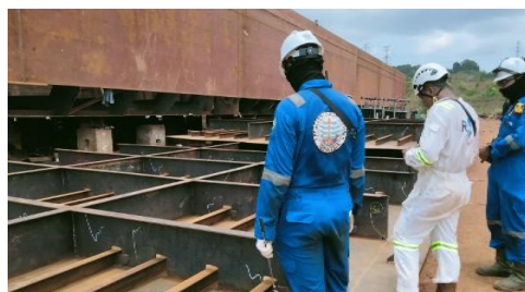
Gambar 2.122. Visual Weld Inspection With RINA Surveyor
