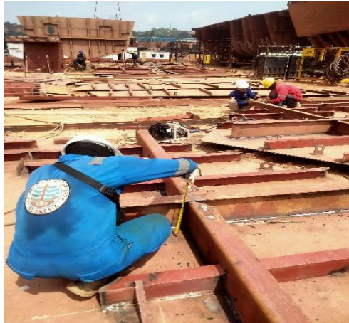
Gambar 2. 39. Fit Up T.Bulkhead
