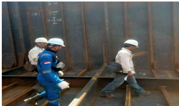
Gambar 2. 112. Visual Weld Inspection
