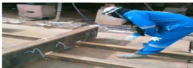
Gambar 2. 217. Visual Welding Inspection
