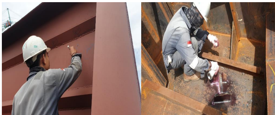
Gambar 2. 254. Visual Welding Inspection and Penetrant Test
