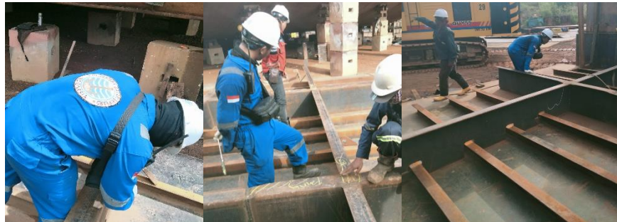
Gambar 2. 195. Visual Welding Inspection
