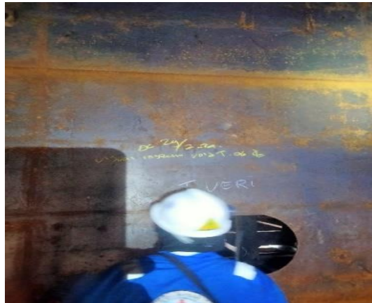
Gambar 2. 45. Visual Weld Inspection Tank
