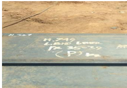
Gambar 2. 44. Visual Weld Inspection
