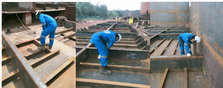
Gambar 2. 177. Visual Weld Inspection
