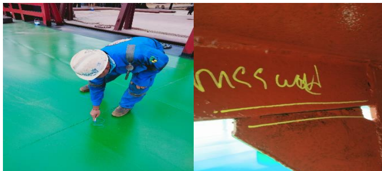
Gambar 2. 171. Final Visual Weld Inspection
