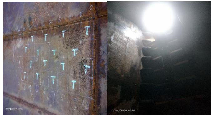
Gambar 2. 66. Air Test Internal Tank
