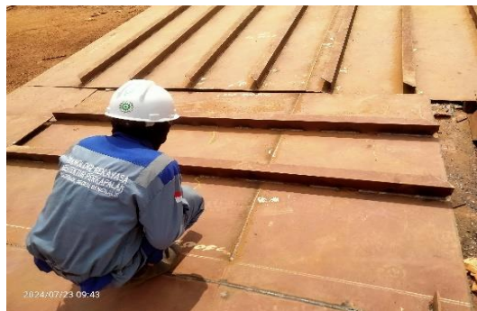
Gambar 2. 30. Visual Weld Inspection T.Bulkhead
