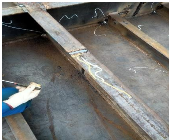
Gambar 2. 40. Visual Weld Inspection T.Bulkhead
