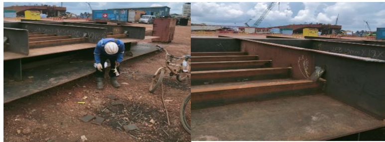
Gambar 2. 182. Visual Weld Inspection
