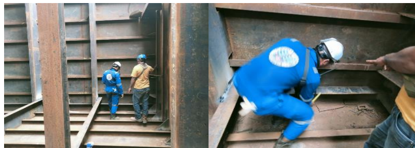
Gambar 2. 202. Fit Up Tank
