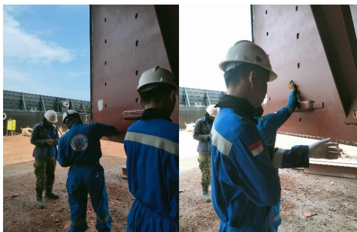
Gambar 2. 133. Final Visual Weld Inspection After Primer Coating
