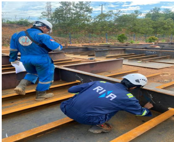
Gambar 2. 101. Visual Weld Inspection With Surveyor
