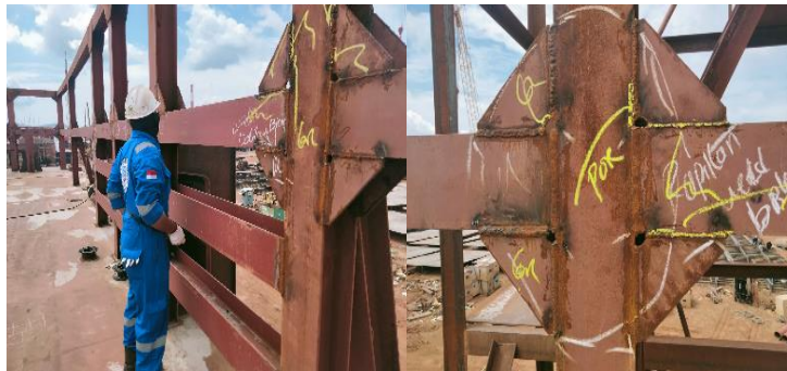
Gambar 2. 198. Visual Welding Inspection
