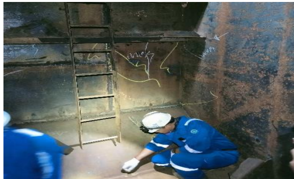
Gambar 2. 126. Visual Weld Inspection Tank
