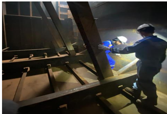
Gambar 2. 118. Visual Weld Inspection Tank
