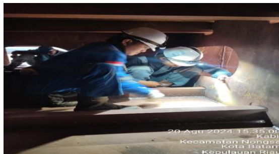
Gambar 2. 95. Visual Weld Inspection Wing Tank
