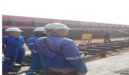
Gambar 2. 52. Visual Weld Inspection Transom After
