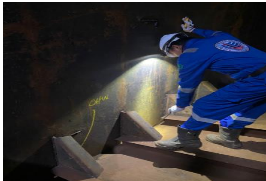
Gambar 2. 98. Visual Weld Inspection Tank
