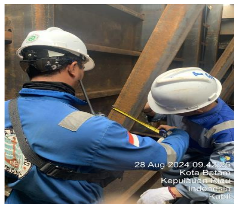
Gambar 2. 114. Fit Up Tank
