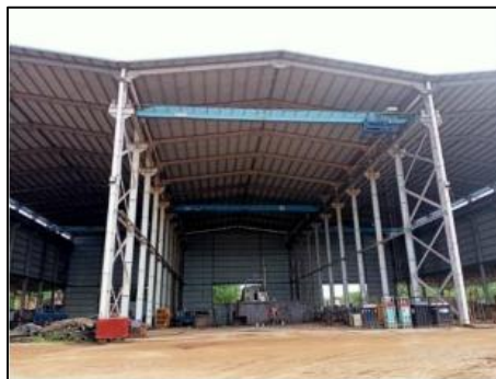
Gambar 1.3 Main Workshop Fabrication
