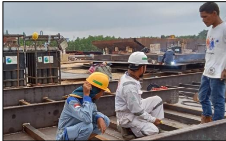
Gambar 2.74 : Proses visual inspect
