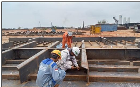
Gambar 2.69 : Proses welding inspection
