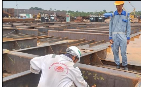
Gambar 2.70 : Proses welding inspection
