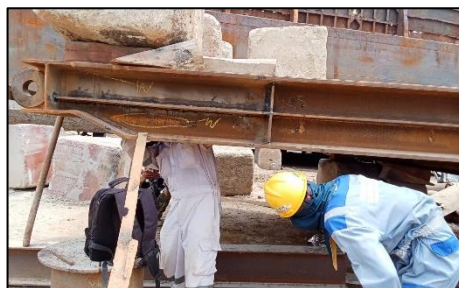
Gambar 2.79 : visual welding ramdor
