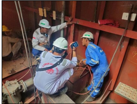
Gambar 2.8 : Proses air test FO tank
