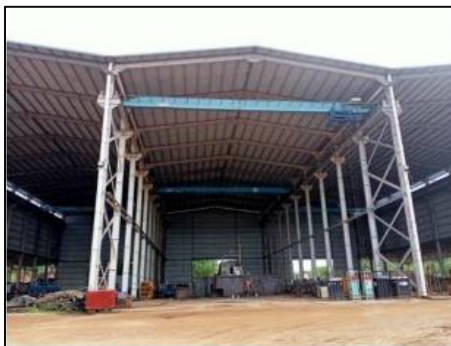
Gambar 1.3 Main Workshop Fabrication
