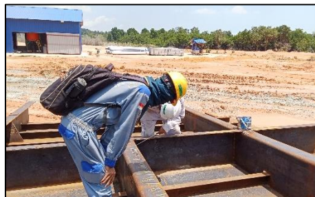
Gambar 2.71 : Proses fit up before welding
