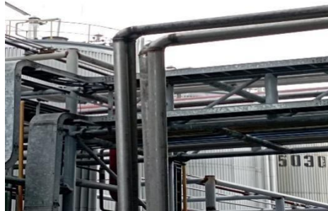
gambar 1 12 penginstalan line air
