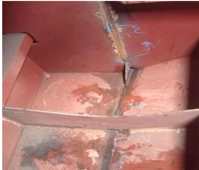
Gambar 2.94 Visual welding inspection
