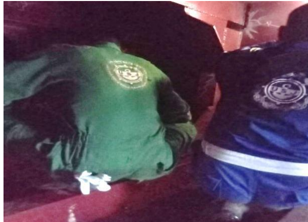
Gambar 2.41 Visual welding inspection
