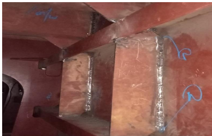
Gambar 2.116 Visual welding inspection
