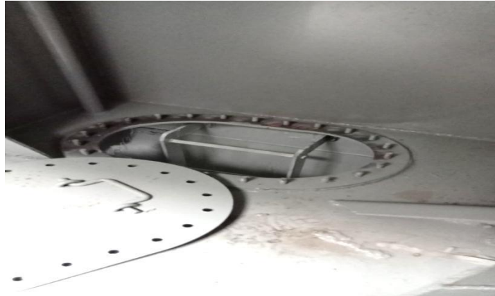
Gambar 2.3 Inspection tangki forepeak
