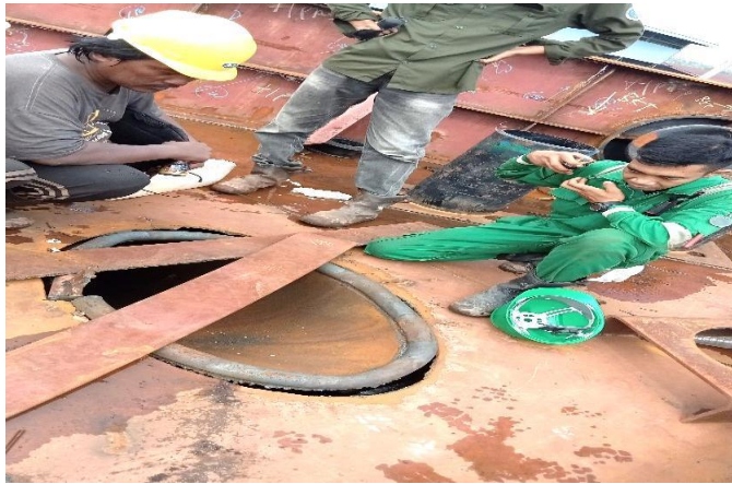
Gambar 2.107 Cek hawse spurling pipe stardboat
