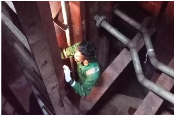
Gambar 2.120 Visual welding inspection
