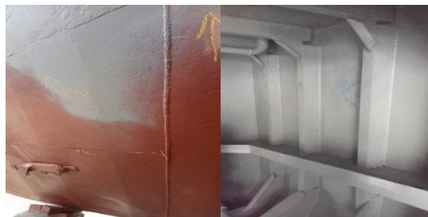
Gambar 2.16 Visual welding inspection
