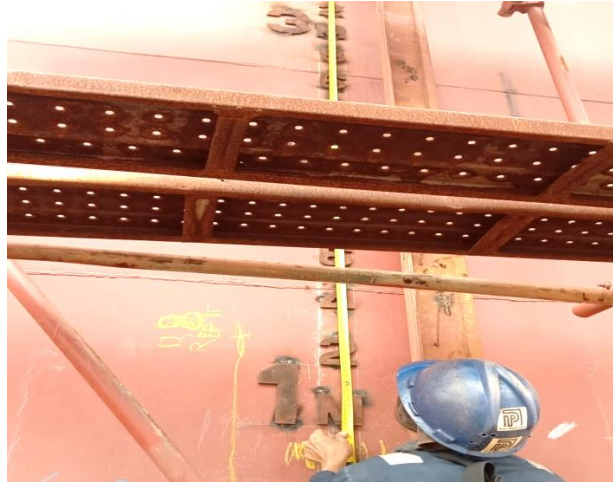
Gambar 2.91 Fit up draft mark
