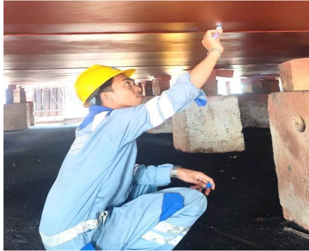
Gambar 2.81 Visual welding inspection
