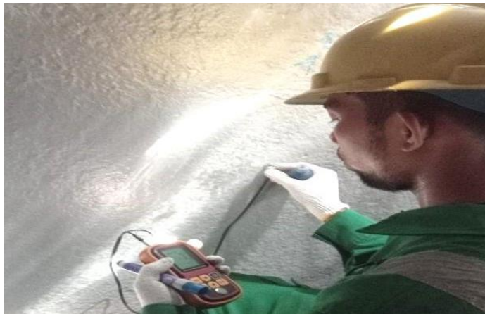
Gambar 2.25 Proses UT Thickness
