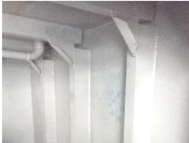
Gambar 2.35 Visual welding inspection
