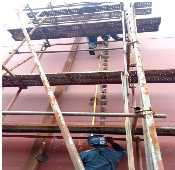
Gambar 2.92 Fit up draft mark
