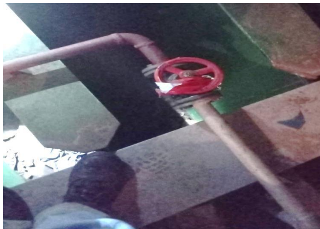
Gambar 2.22 Air test pipe ows
