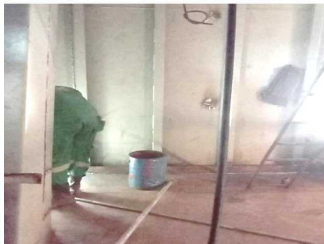
Gambar 2.28 Visual welding inspection
