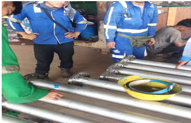
Gambar 2.32 Visual welding inspection
