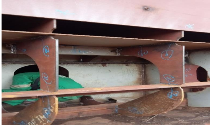
Gambar 2.109 Visual welding inspection
