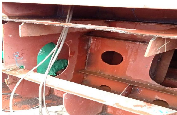
Gambar 2.106 Visual welding inspection
