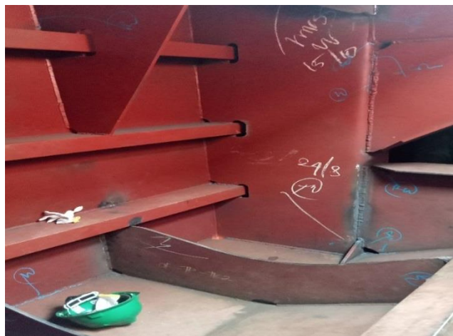
Gambar 2.118 Visual welding inspection
