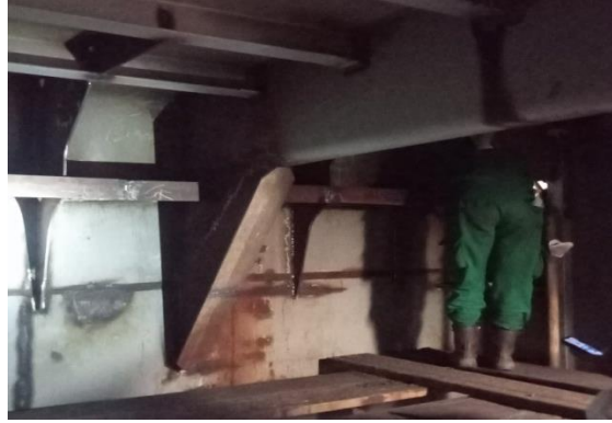
Gambar 2.135 Visual welding inspection
