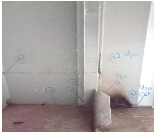
Gambar 2.90 Visual welding inspection
