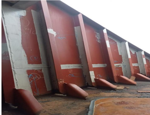
Gambar 2.89 Visual welding inspection
