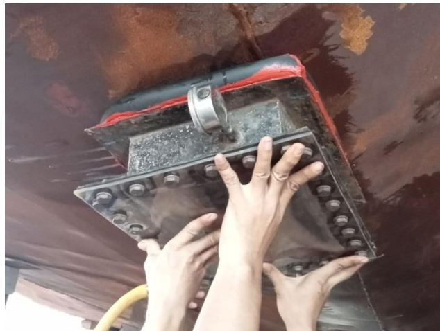
Gambar 2.122 Vacum test
