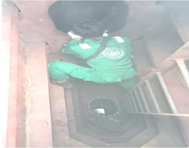
Gambar 2.51 Visual welding inspection
