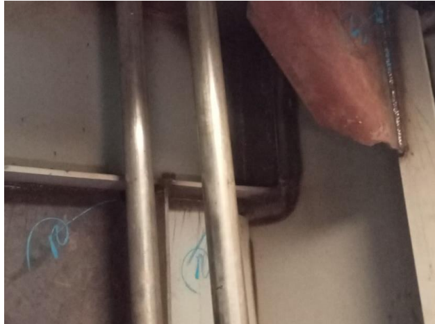
Gambar 2.129 Visual welding inspection
