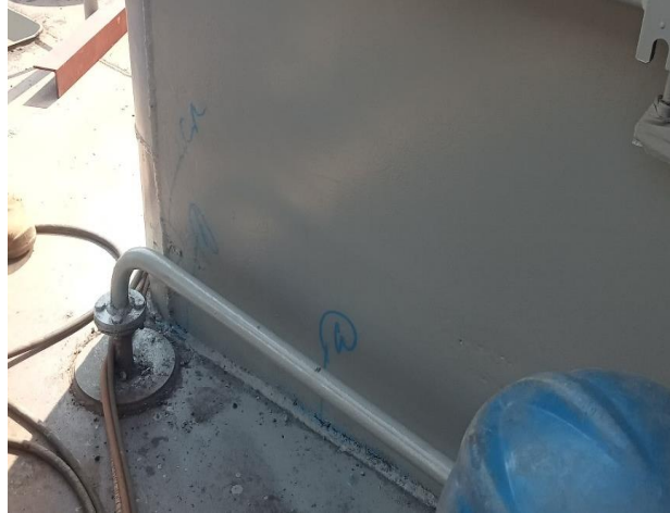
Gambar 2.131 Visual welding inspection
