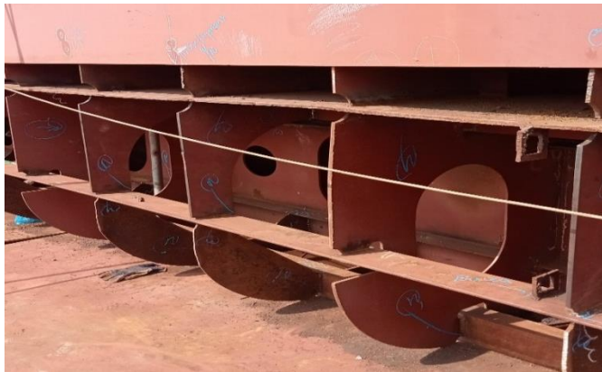
Gambar 2.110 Visual welding inspection
