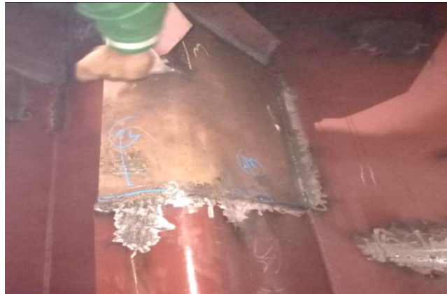
Gambar 2.33 Visual welding inspection
