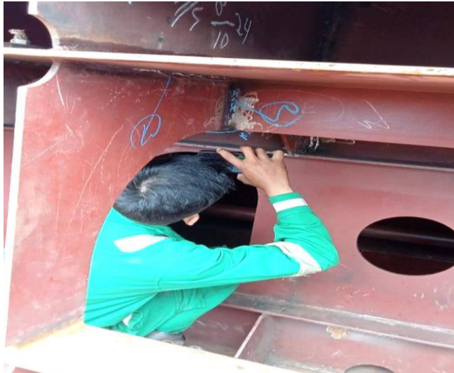
Gambar 2.105 Visual welding inspection
