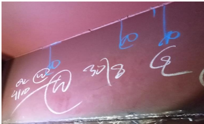
Gambar 2.126 Visual welding inspection
