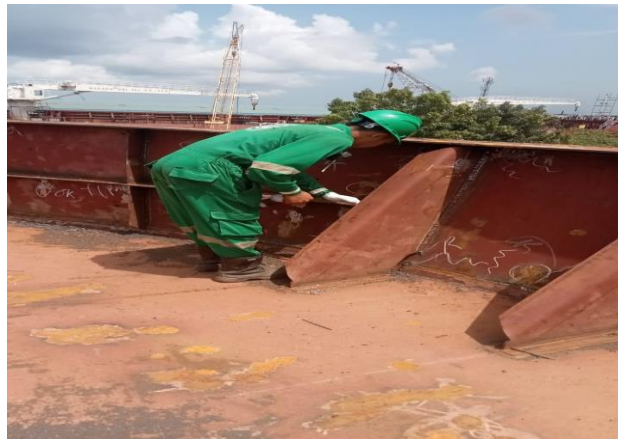
Gambar 2.48 Visual welding inspection
