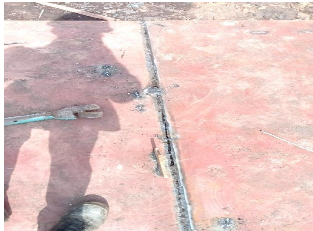
Gambar 2.64 Inspection bevel
