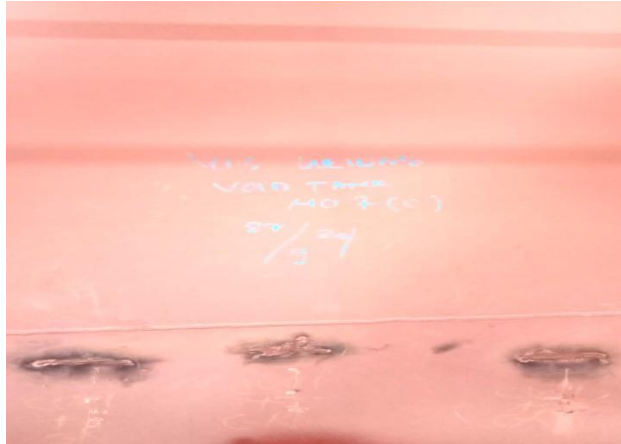
Gambar 2.75 Visual welding inspections
