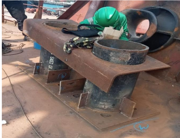
Gambar 2.127 Visual welding inspection
