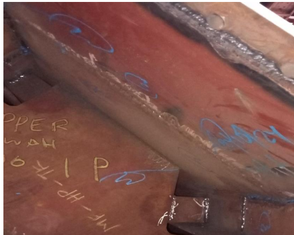
Gambar 2.134 Visual welding inspection
