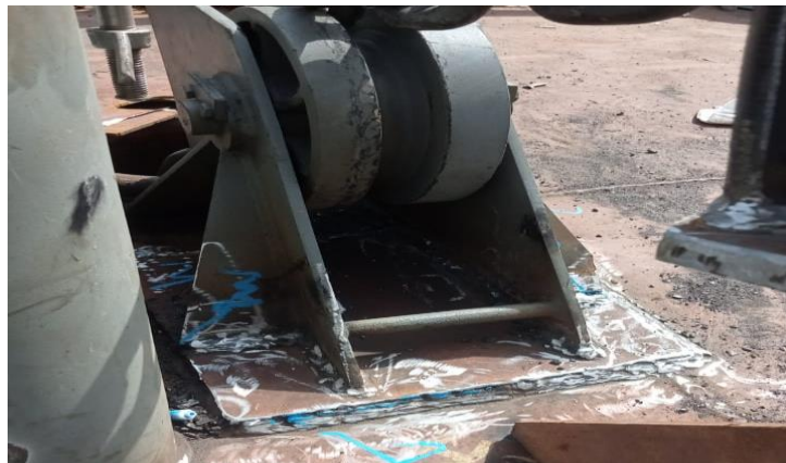
Gambar 2.26 Visual welding inspection
