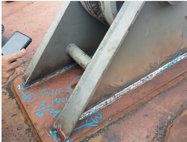
Gambar 2.87 Visual welding inspection
