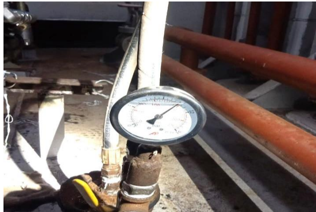
Gambar 2.95 Air test pipe
