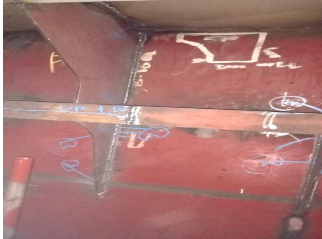
Gambar 2.97 Visual welding inspection
