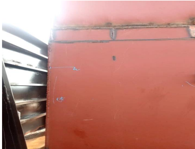
Gambar 2.65 Visual welding inspection
