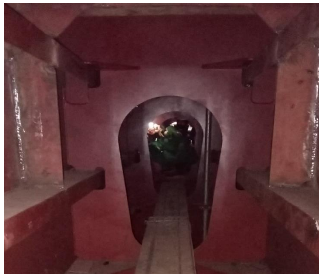
Gambar 2.112 Visual welding inspection
