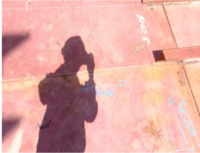
Gambar 2.73 Inspection web frame
