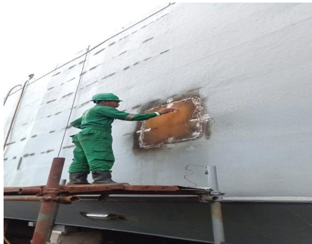
Gambar 2.52 Inspection gouging
