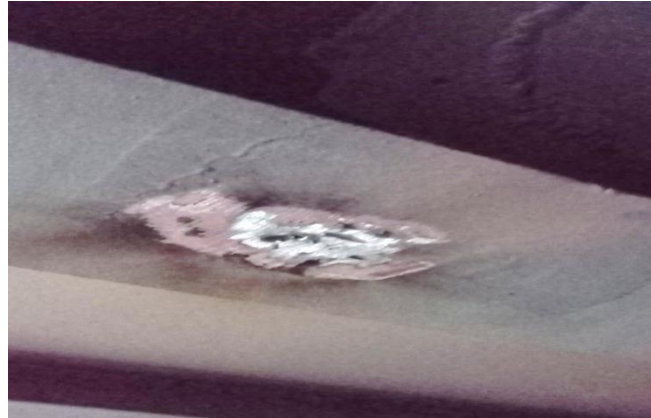
Gambar 2.13 Visual welding inspection
