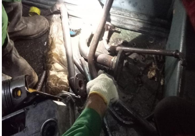
Gambar 2.121 Inspection pipa kuling
