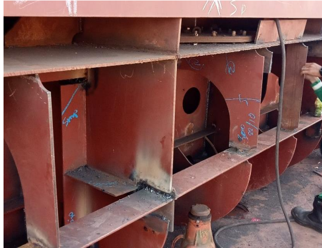
Gambar 2.111 Visual welding inspection
