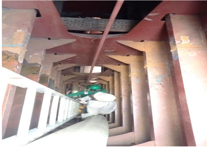
Gambar 2.71 Visual welding inspection
