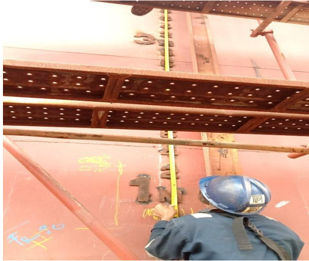
Gambar 2.77 Fit up draft mark
