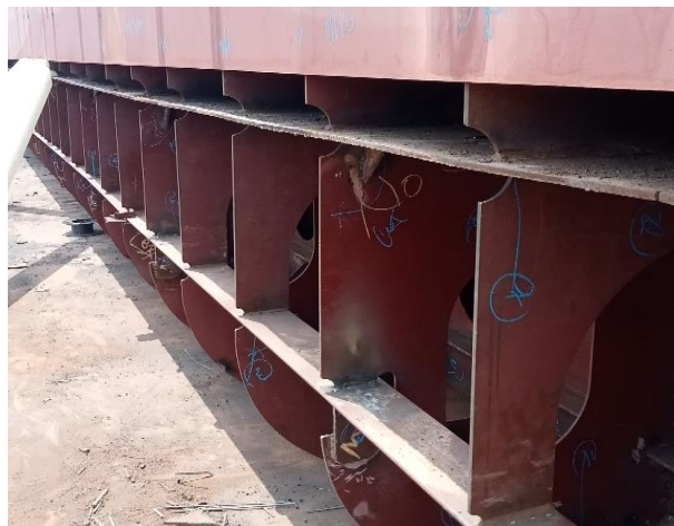
Gambar 2.128 Visual welding inspection
