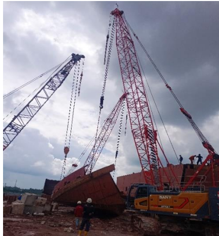
Gambar 2. 6 Erection forepeak barge no 026
