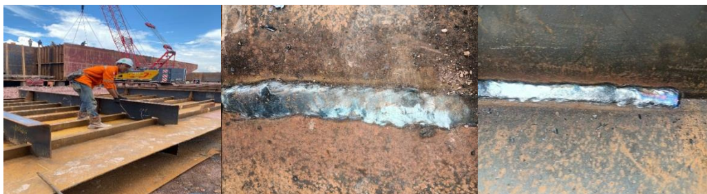
Gambar 3. 18 pengecekan area marking
