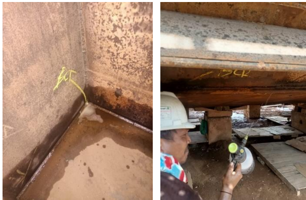
Gambar 2. 29 peroses Air Parasure Test
