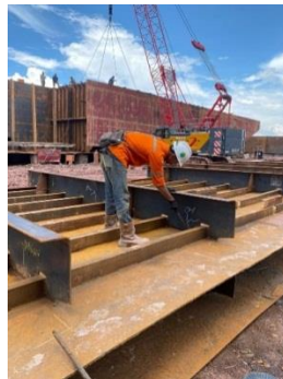
Gambar 2. 76 visual Inspect side shell
