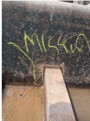
Gambar 2. 73 visual inspect tanki
