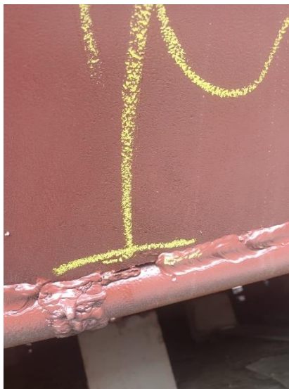
Gambar 2. 72 pengecekan lubar air
