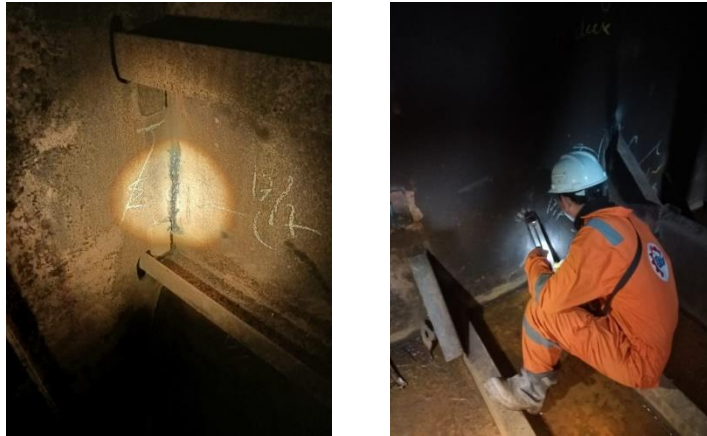
Gambar 2. 22 Visual Inspect tanki
