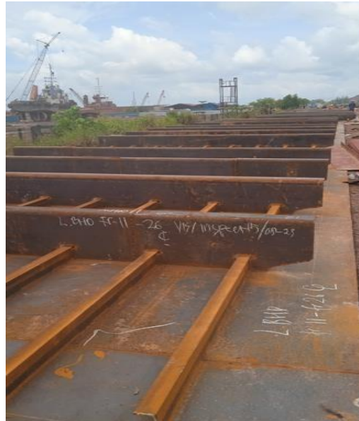
Gambar 2. 34 Visual Inspect L.bhd
