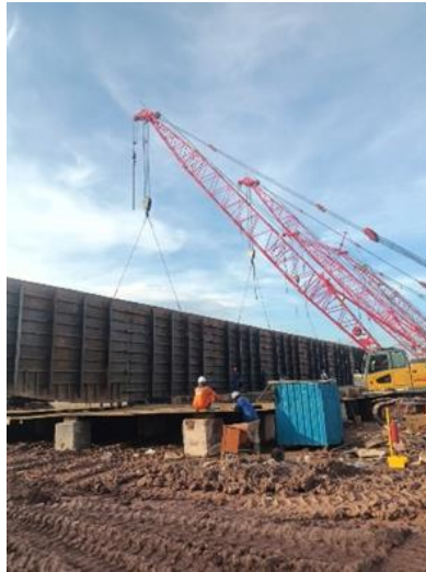
Gambar 2. 50 Erection L.bhd
