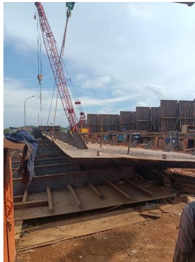
Gambar 2. 37 proses Erection L.bhd
