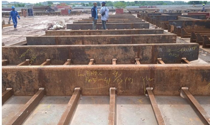
Gambar 2. 43 visual inspect L.bhd
