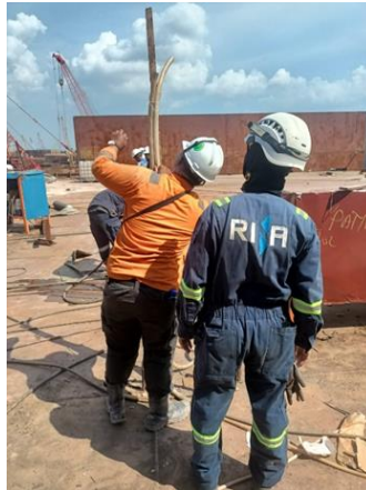
Gambar 2. 60 proses air test external
