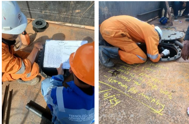
Gambar 2. 1 Visual inspect tanki
