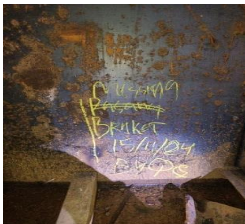
Gambar 3. 10 missing bracket
