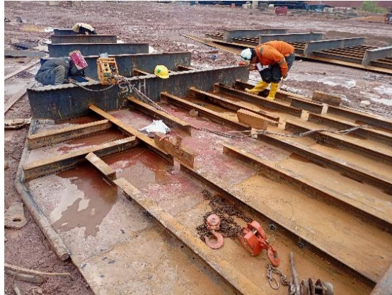
Gambar 2. 52 Visual welding inspection
