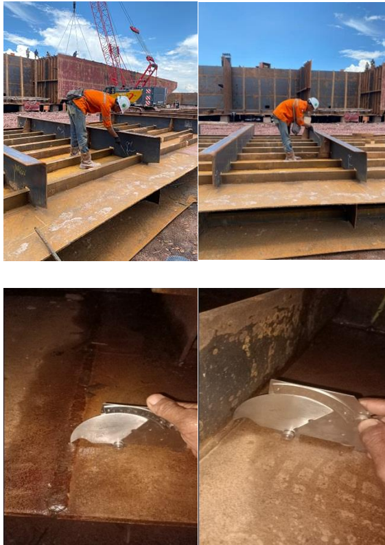
Gambar 3. 13 Visual inspect welding
