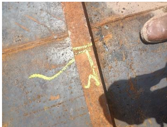
Gambar 3. 16 crack
