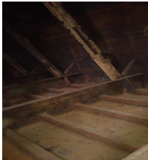
Gambar 2. 21 pengecekan rembesan air
