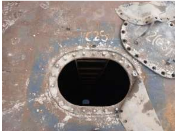
Gambar3.2membuka main hole
