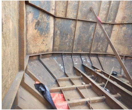
Gambar 2, 9 visual welding inspection
