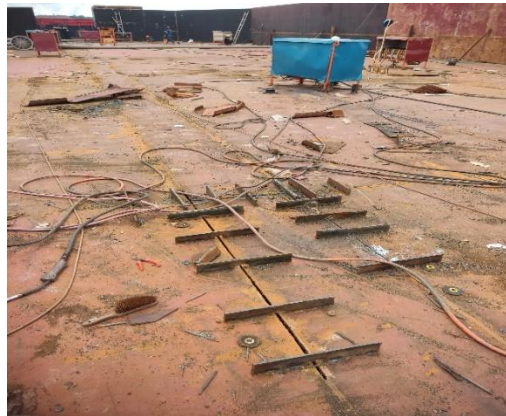
Gambar 2. 44 Repair main deck
