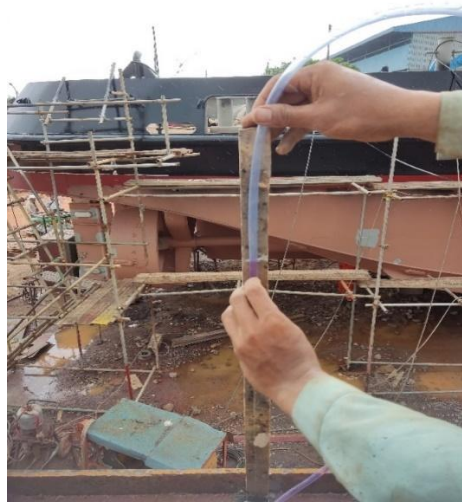
Gambar 2, 11 levelling raised deck
