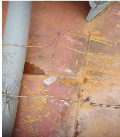
Gambar 2. 30 Visual inspeksi main deck
