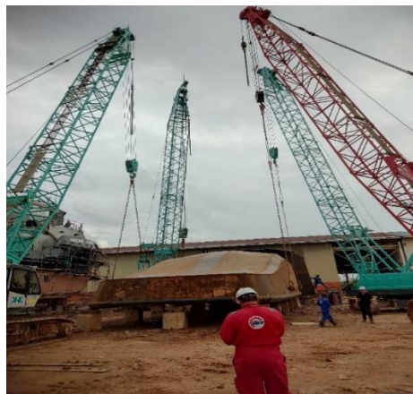
Gambar 2, 10 lifting turning
