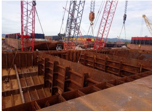
Gambar 2. 36 Bending ceruk Buritan
