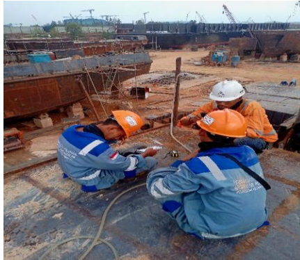
Gambar 2, 5 Leveling raised deck
