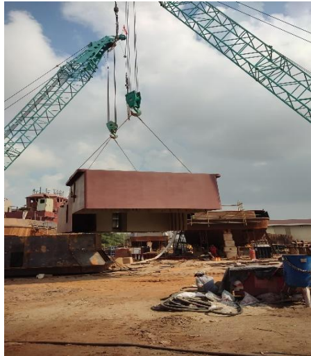
Gambar 2. 40 lifting turning
