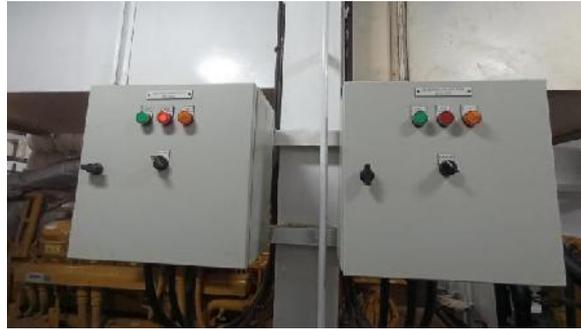
Gambar 3. 12 Panel ballast/bilge pump
