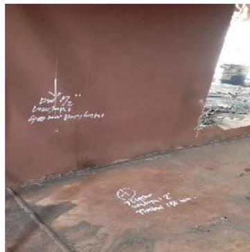
Gambar 2. 88 Marking jalur pipa
