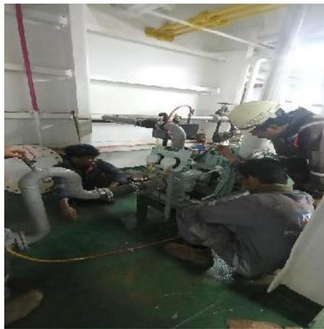
Gambar 2. 82 Pengecekan *emergency fire pump*
