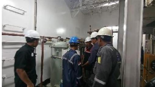
*Gambar 2. 102 Proses Commissioning oily bilge separator*
