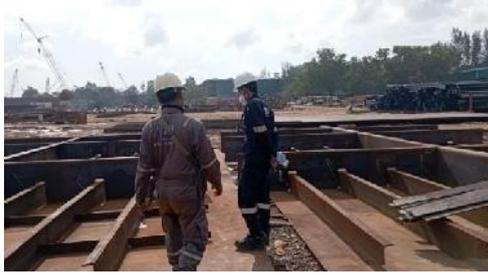
Gambar 2. 6 *Inspect Welding terhadap panel main deck*
