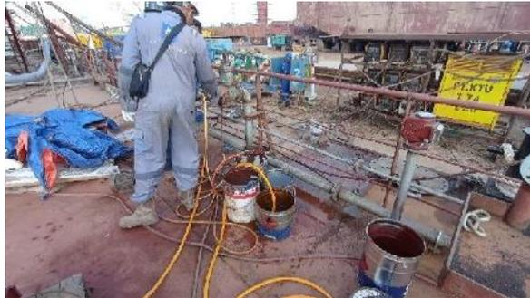
*Gambar 2. 54 Proses Hydro test pipa hydrant*
