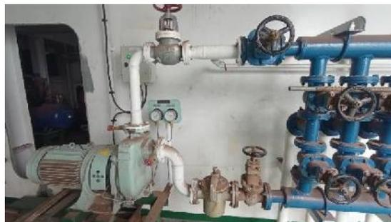
Gambar 2. 71 Fresh water transfer pump
