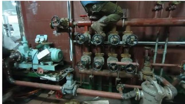
Gambar 2. 59 Perpipaan Fuel Oil Crane Barge
