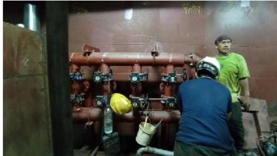
Gambar 2. 46 manifold cabang ballast
