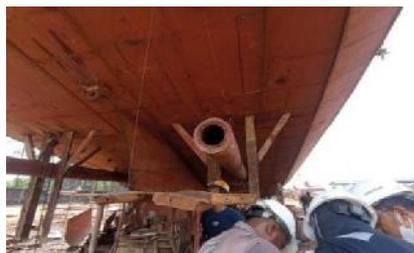
*Gambar 2. 20 Alignment test stern tube tugboat*
