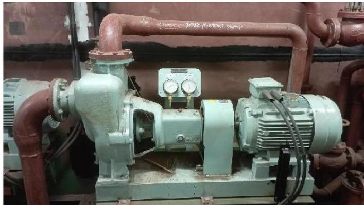
Gambar 2. 72 Ballast transfer pump
