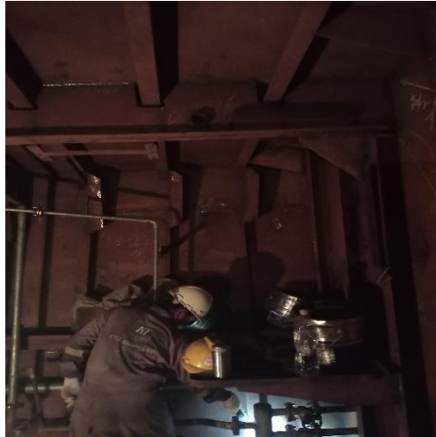
Gambar 2. 51 Inspect dibagian Engine Room
