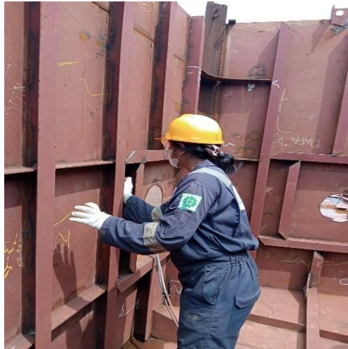
Gambar 2. 52 Inspect welding deck house
