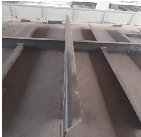
Gambar 2. 10 Inspect welding panel main deck.
