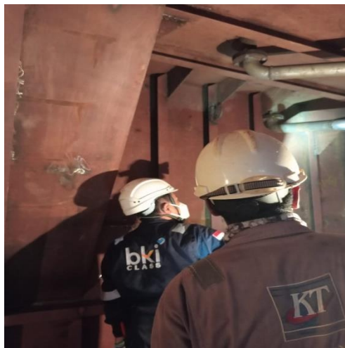
Gambar 2. 47 Inspect welding terhadap tangki
