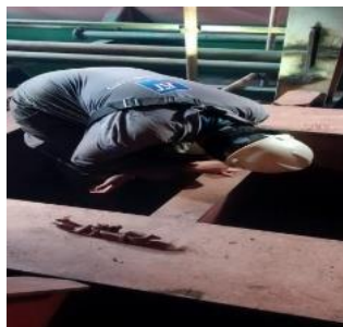
Gambar 2. 65 proses inspect welding
