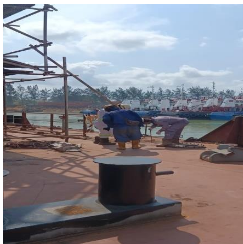
Gambar 2. 30 Inspect welding bagian main deck
