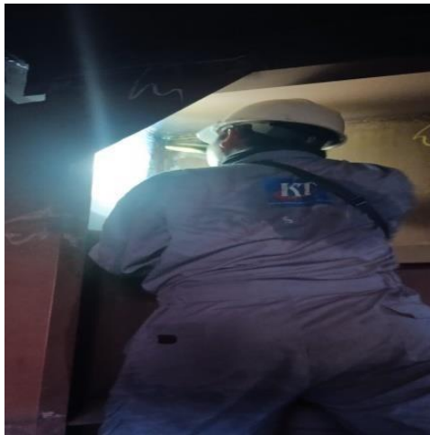
Gambar 2. 34 inspect welding tangki void crane
