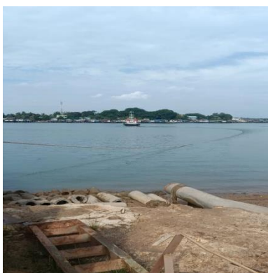
Gambar 2. 68 Proses bollard test
