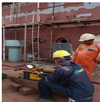
Gambar 2. 54 Proses hydro test
