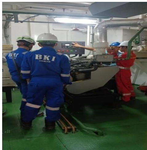
Gambar 2. 71 proses load test
