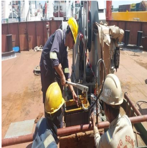
Gambar 2. 53 Proses hydro test
