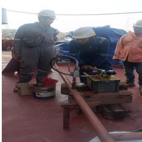
Gambar 2. 61 proses hydro test
