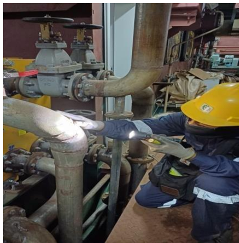
Gambar 2. 46 proses hydro test
