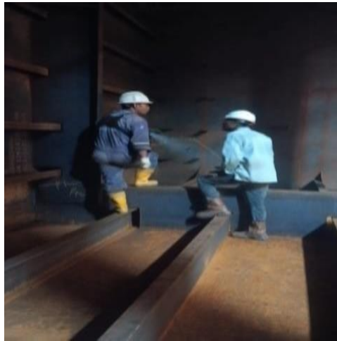
Gambar 2. 4 proses inspect welding and scantling
