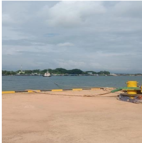
Gambar 2. 62 proses bollard test
