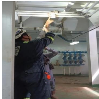
Gambar 2. 60 Proses inspect welding
