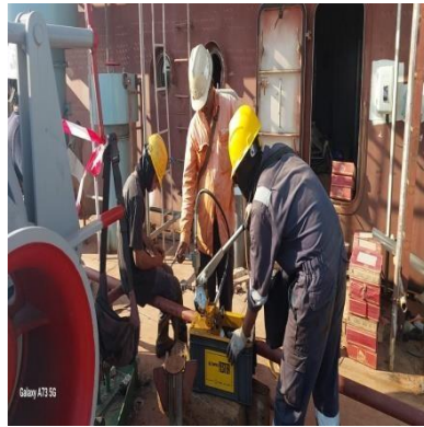
Gambar 2. 55 Proses hydro test
