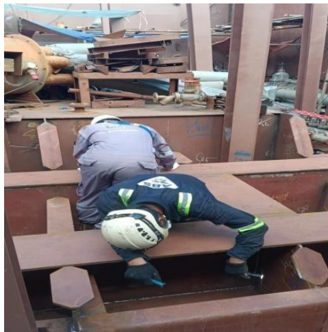
Gambar 2. 51 proses inspect welding
