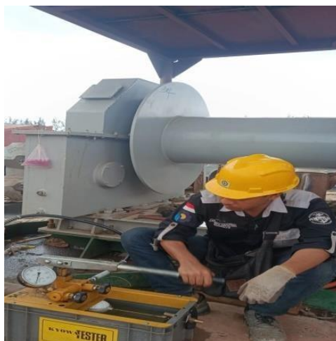
Gambar 2. 57 pengecekan engine room
