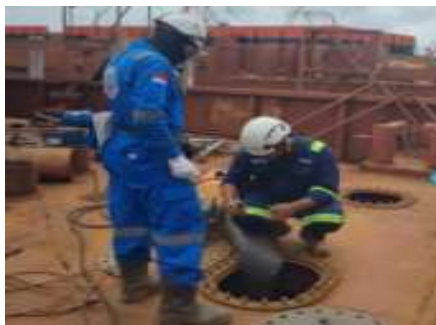
Gambar 2. 83 Visual welding tank Inspection
