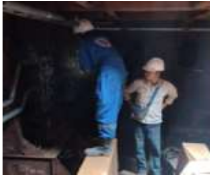
Gambar 2. 84 Visual welding tank Inspection
