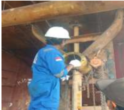
Gambar 2.9 Pengecekan Stress Tube
