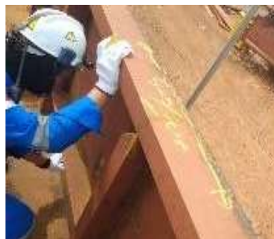
Gambar 2. 6 visual welding inspection (SMAW)
