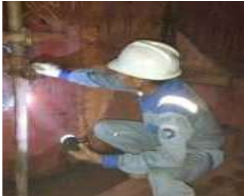
Gambar 2. 110 Air Pressure Test Eksternal
