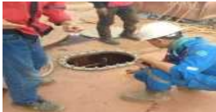
Gambar 2. 123 Air Pressure Test Eksternal
