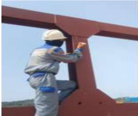
Gambar 2. 92 Air Pressure Test Eksternal
