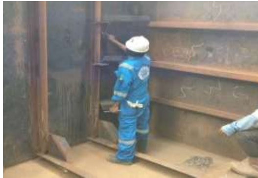
Gambar 2. 62 Visual welding tank
