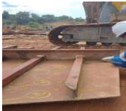
Gambar 2. 3 Visual Welding Inspection
