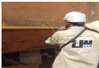
Gambar 2. 23 Proses Leveling Draft
