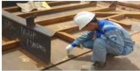
Gambar 2. 115 Visual welding Inspection
