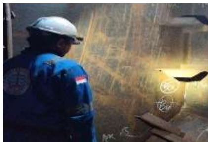
Gambar 2. 22 Visual welding tank
