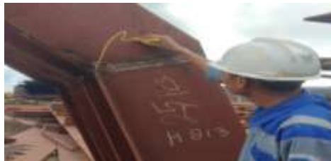
Gambar 2. 113 visual welding inspection
