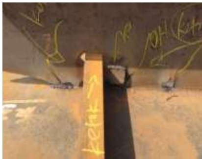
Gambar 2. 12 Visual welding Inspect
