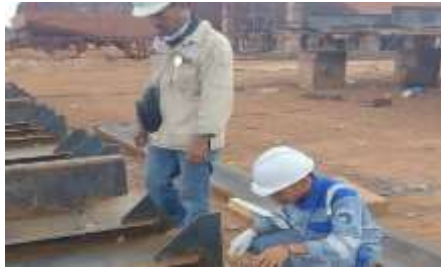
Gambar 2. 28 Visual welding inspection
