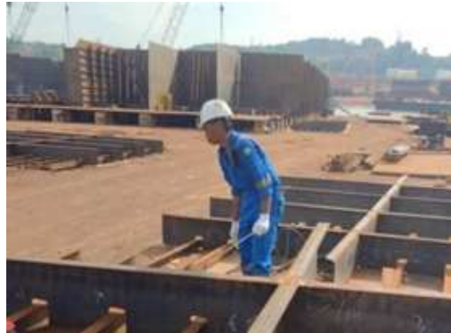
Gambar 2. 60 Visual welding inspection
