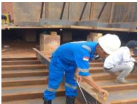
Gambar 2. 36 Visual Welding Inspection
