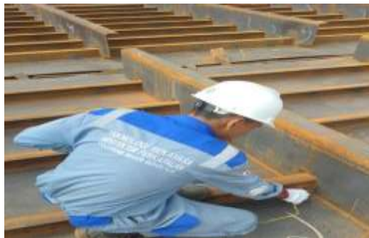
Gambar 2. 61 Visual welding inspection
