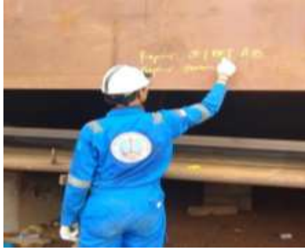
Gambar 2. 33 Visual Welding Inspection
