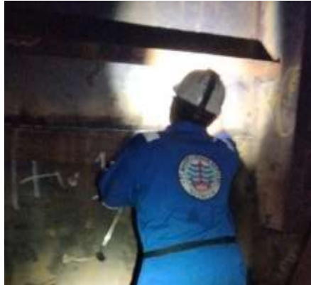
Gambar 2. 48 Visual Inspect welding
