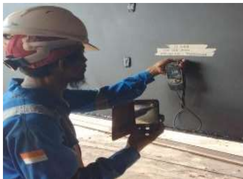
Gambar 2. 47 pengecekan Thickness Coating
