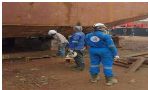
Gambar 2. 121 Visual Gouging Inspection
