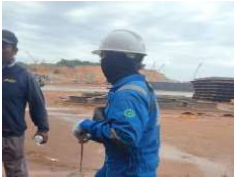
Gambar 2. 50 Visual Inspect welding
