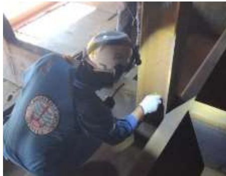
Gambar 2. 24 Visual inspection tank
