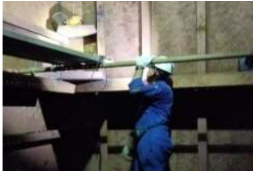
Gambar 2. 54 Visual welding tank
