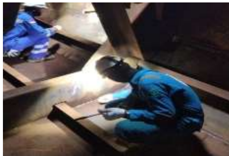
Gambar 2. 120 Visual Welding tank inspection
