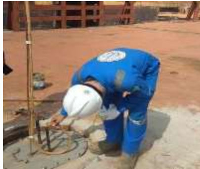
Gambar 2. 71 Air Pressure Test Internal
