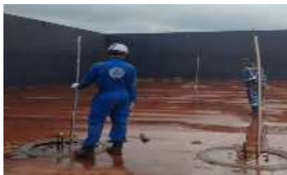
Gambar 2. 32 Air Pressure Test Eksternal
