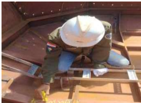
Gambar 2. 99 Visual welding Inspection
