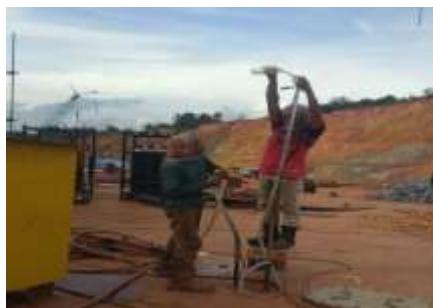
Gambar 2. 119 Air pressure test eksternal
