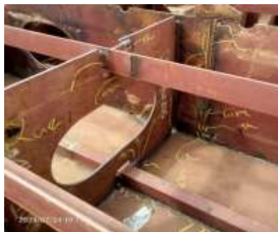
Gambar 2. 15 Visual welding inspection
