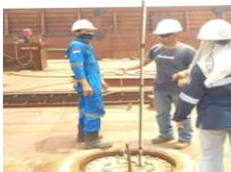
Gambar 2. 72 Air Pressure Test Internal
