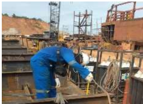
Gambar 2. 55 Leveling Bottom
