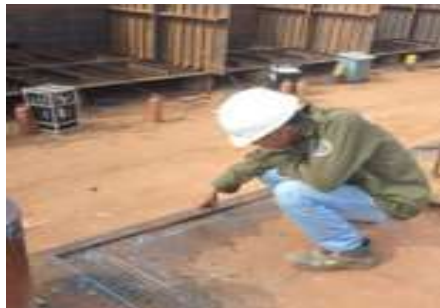
Gambar 2. 91 Visual welding Inspection
