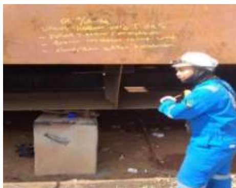
Gambar 2. 25 Visual welding tank
