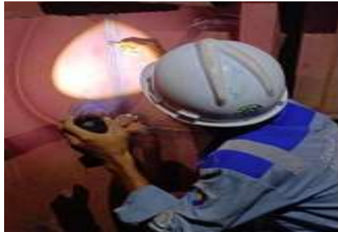
Gambar 2. 58 Visual welding tank
