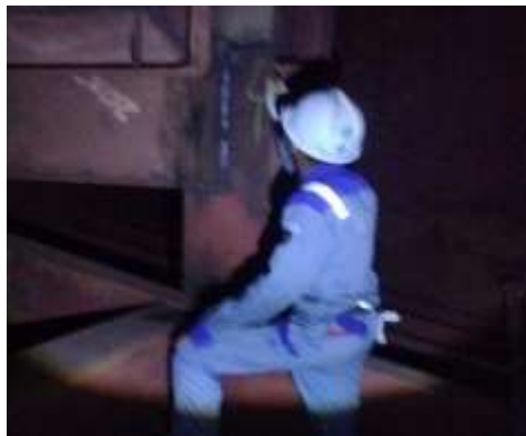
Gambar 2. 95 visual welding tank inspection
