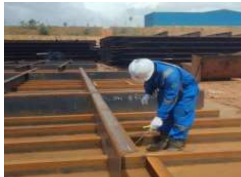
Gambar 2. 38 Visual welding Inspection
