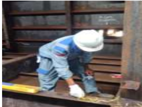
Gambar 2. 64 Visual welding tank Inspection
