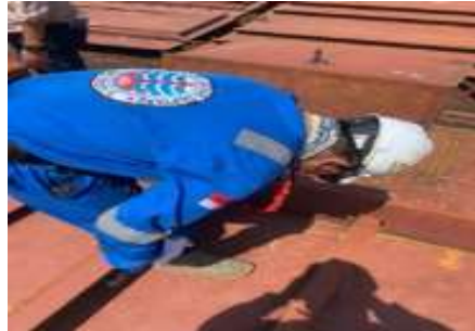
Gambar 2. 65 Visual welding Inspection
