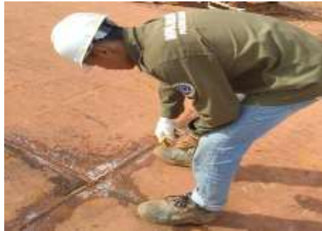
Gambar 2. 98 Air Pressure Test Eksternal
