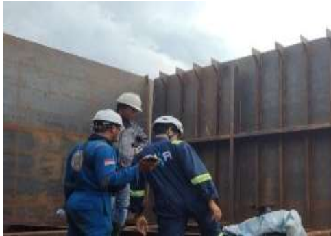
Gambar 2. 35 Visual Welding inspection
