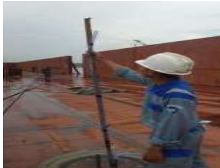
Gambar 2. 104 Air Pressure Test Eksternal
