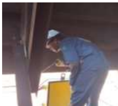
Gambar 2. 81 Visual welding tank Inspection
