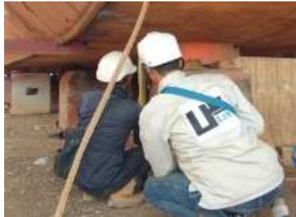
Gambar 2. 21 Proses levelling Bottom
