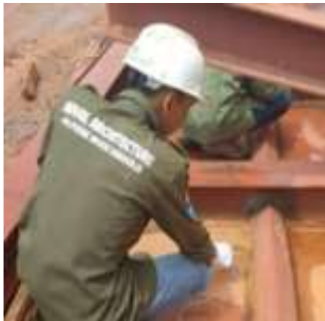
Gambar 2. 97 Visual welding Inspection
