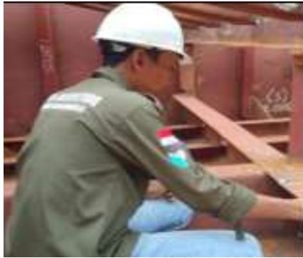
Gambar 2. 88 Visual welding Inspection
