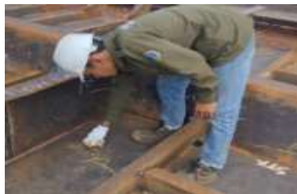
Gambar 2. 79 Visual welding Inspection
