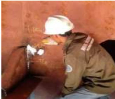
Gambar 2. 73 Visual welding tank Inspection
