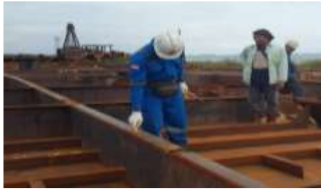
Gambar 2. 117 Visual welding Inspection
