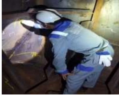
Gambar 2. 100 Visual welding Inspection
