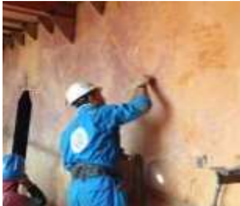
Gambar 2. 108 Visual Welding Inspection
