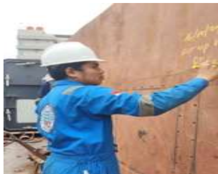
Gambar 2. 85 Visual welding Inspection
