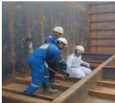
Gambar 2. 34 Visual Welding inspection
