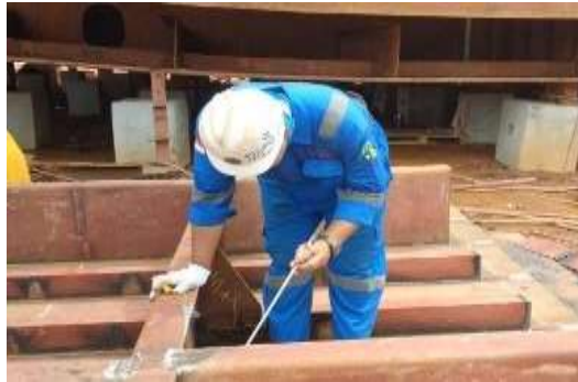
Gambar 2. 46 Visual Inspect welding
