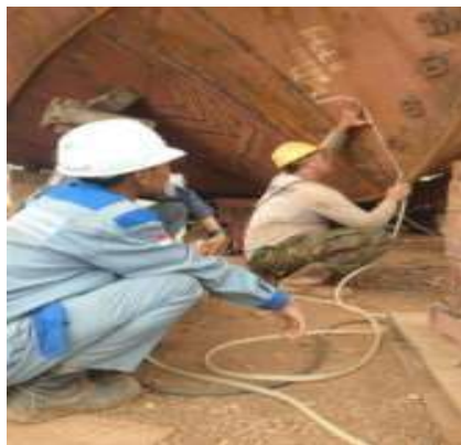
Gambar 2. 105 Leveling Bottom
