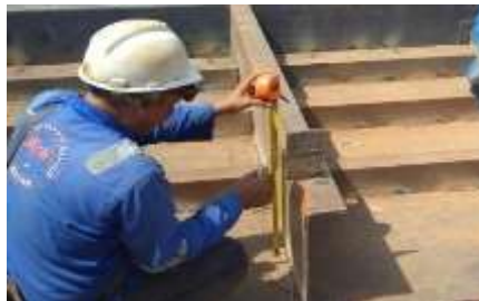
Gambar 2. 18 Proses Leveling Deck
