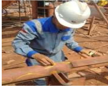
Gambar 2. 122 Visual welding Inspection
