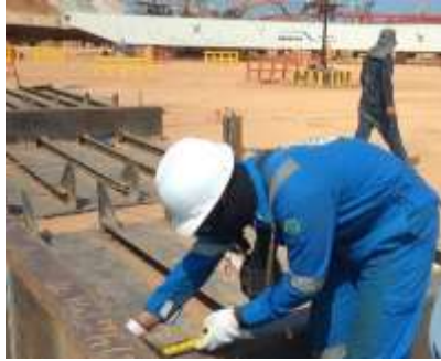
Gambar 2. 19 Visual Inspection Welding
