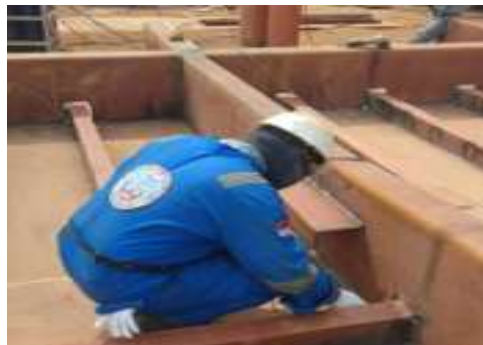
Gambar 2. 49 Visual Inspect welding
