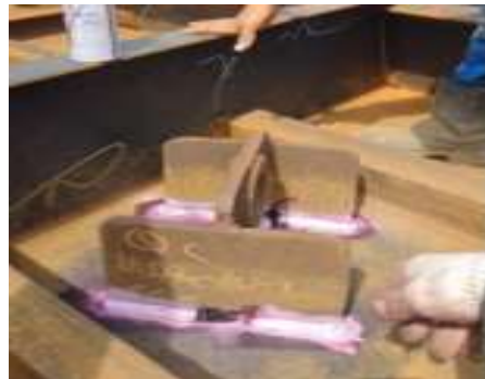
Gambar 2. 53 Penetran test inspection
