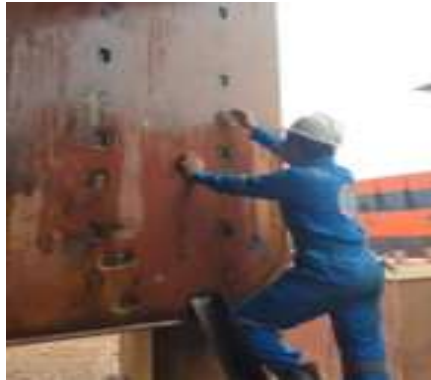
Gambar 2. 86 Air Pressure Test Eksternal
