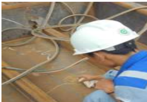
Gambar 2. 45 Visual Inspection Welding
