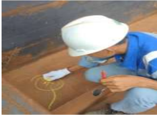
Gambar 2. 66 Visual welding Inspection
