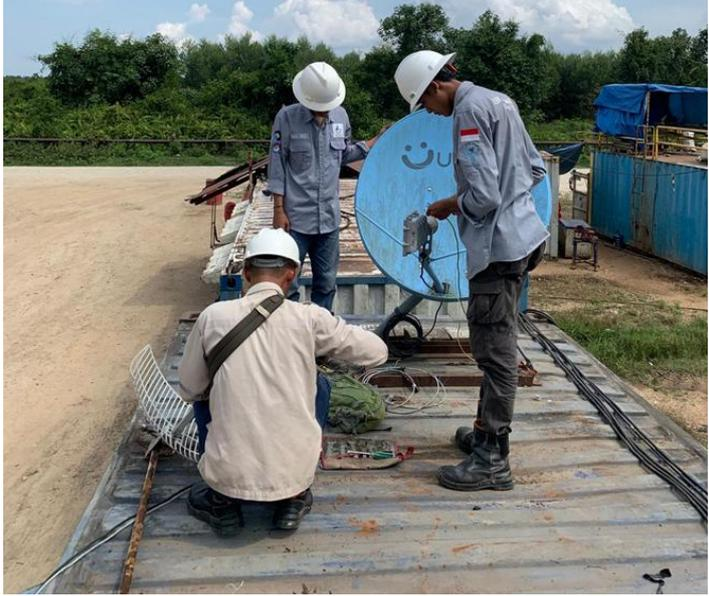
A photograph showing three workers on a metal platform, likely the deck of a boat, installing a VSAT antenna. One worker is kneeling in the foreground, another is standing and working on the antenna, and a third is standing in the background. The antenna is a large, circular, blue dish. The background shows a sandy area and some greenery. |
