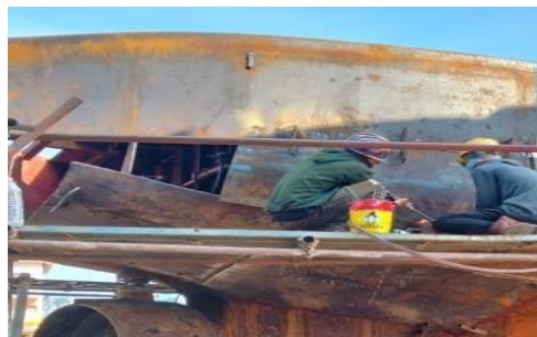
Gambar 2.7 Replaiting plate buritan
