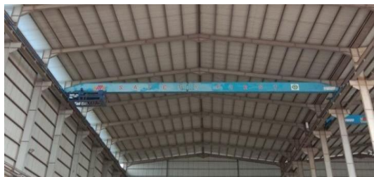
Gambar 1.6 Overhead Crane
