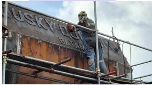
Gambar 2.15 Pemasangan port register TB.Dusky Dolphin
