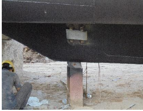
Gambar 2.37 Install zinc anode new
