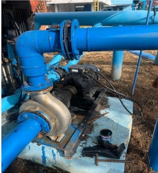
Gambar 3 7 pompa intake
