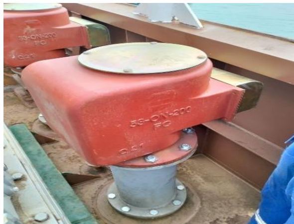
Gambar 2.45 Air Vent Head
