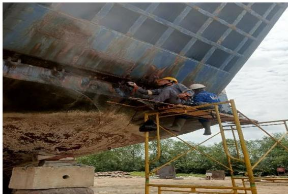
**Gambar 2.22** *Penetrant Test bagian Engsel Ramdoor*
