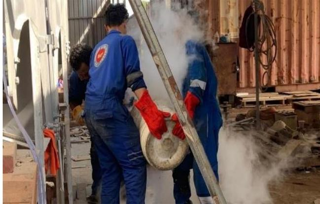
Gambar 3 7 pemasangan busing shaft
