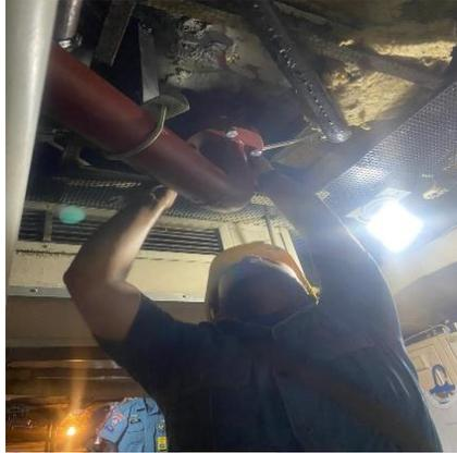
*Gambar 2.28 Pemasangan Pipa Sewage*
