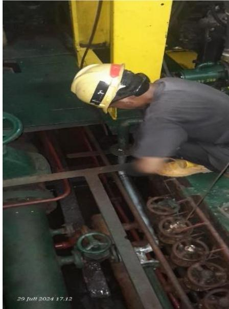
*Gambar 2.14 Mengganti Pipa SW Cooling Air*
